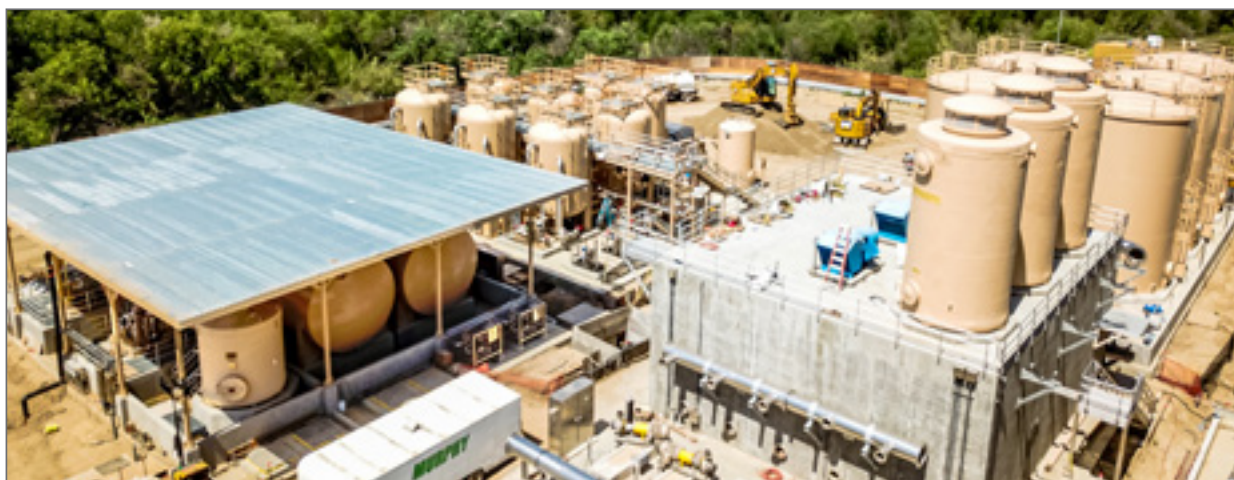
Valencia WRP's Advanced Water Treatment Facility under construction
