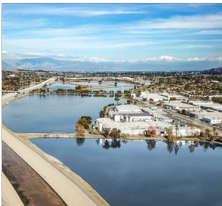
The Rio Hondo Coastal Spreading Grounds uses reclaimed water to replenish groundwater.
