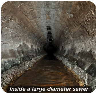
Inside a large diameter sewer
