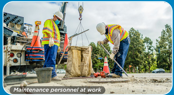
Maintenance personnel at work
