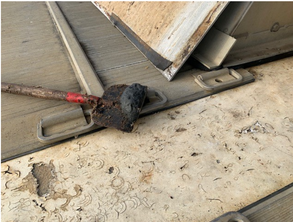
Figure 2: 9-8-2021 photo of a large grease ball at the JWPCP headworks bar screens. Note hoe for scale.
