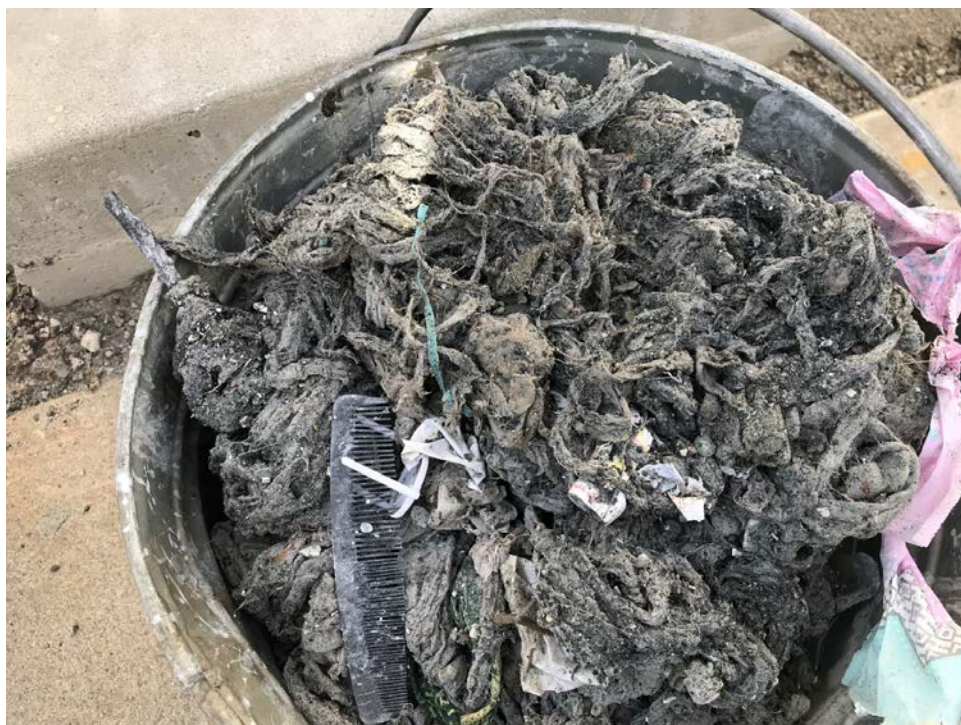
Figure 2: "Rags" removed from the J.O. 'E' Unit 3 trunk sewer line in a bucket at the Compton field office on 1-19-2021.
