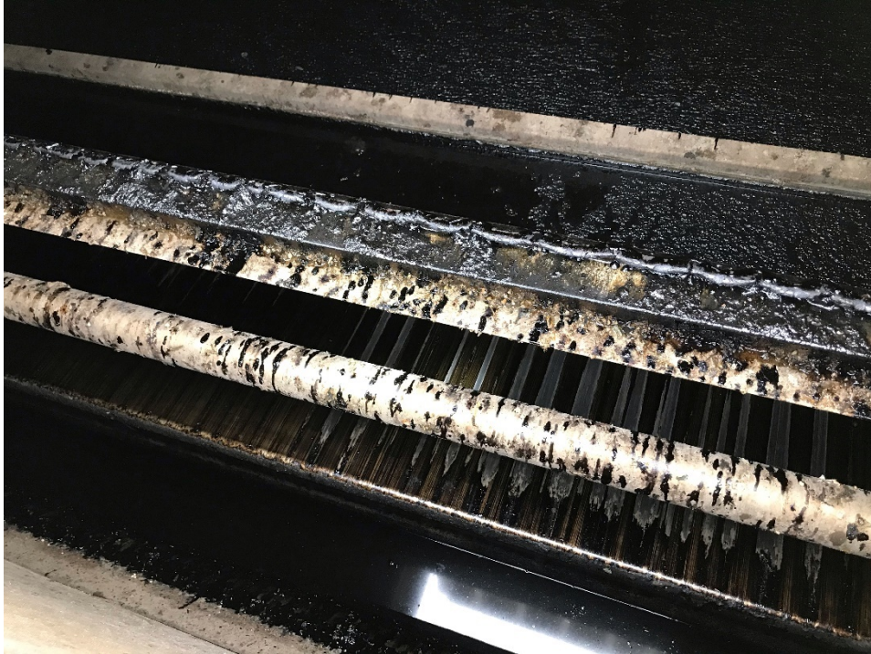
Figure 2: Black oil globules on the JWPCP E1 skimmings trough on the morning of 2-9-2021.
