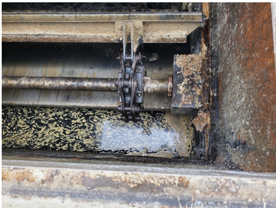
Figure 3: Oily material in JWPCP North Skimmer trough on 4-14-2021 at 1300 hours.
