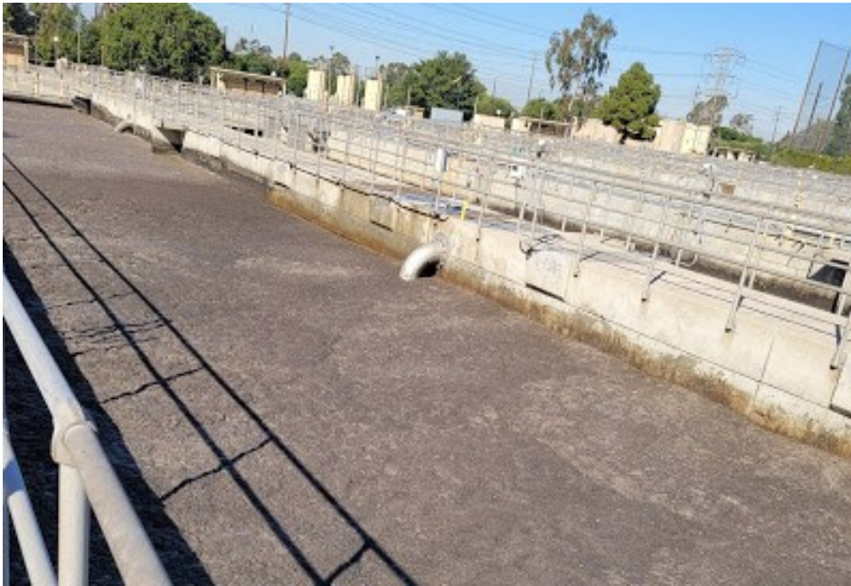
Figure 7: 2-18-2021 excessive foam in aeration tank at LCWRP at 0730 hours.
