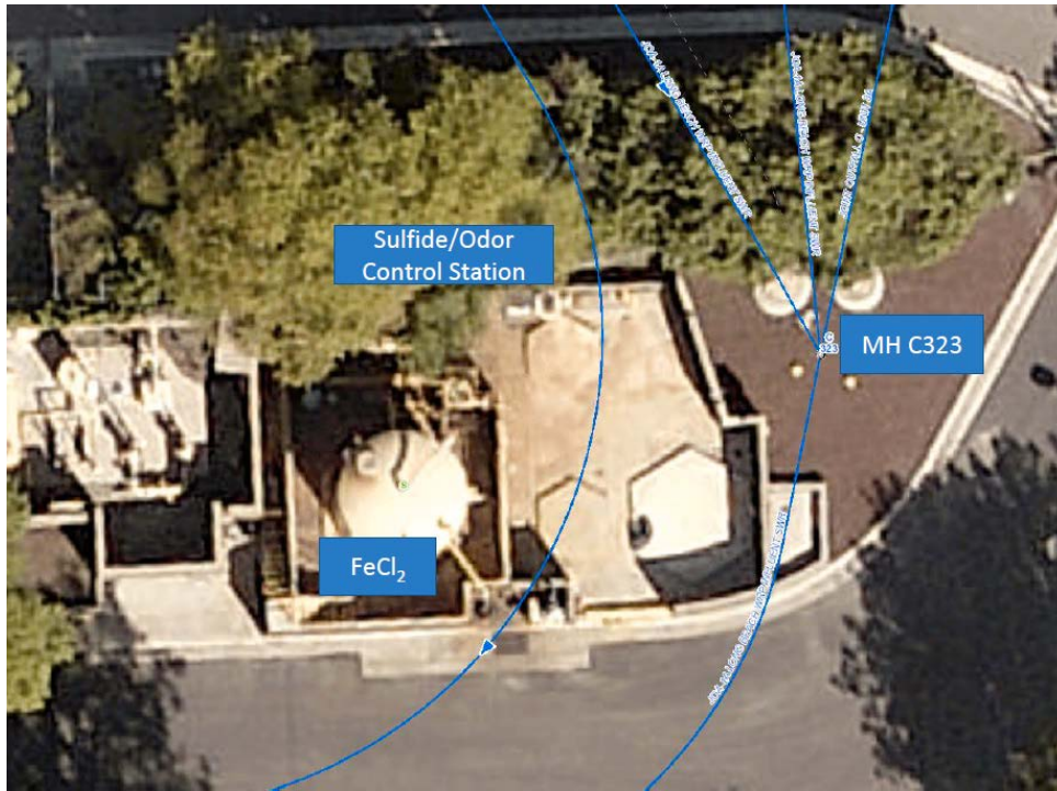
Figure 7: Districts' GIS screen grab photo showing the ferrous chloride addition system at the Long Beach WRP odor control station.
