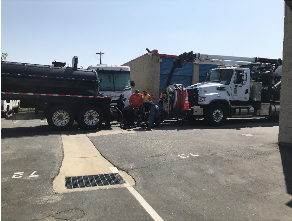
Figure 10: Cleaning the local line on 3-30-2021.
