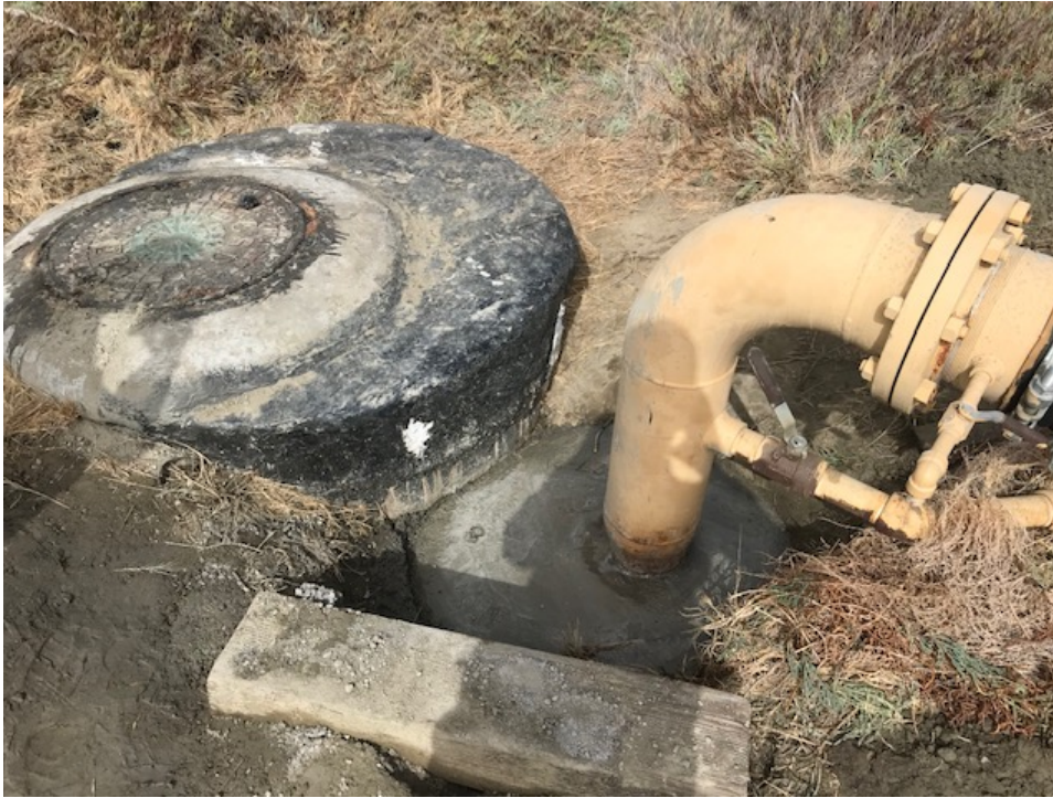
Figure 14: 8-14-2021 work showing the finished concrete repair work at MH 03 0556.
