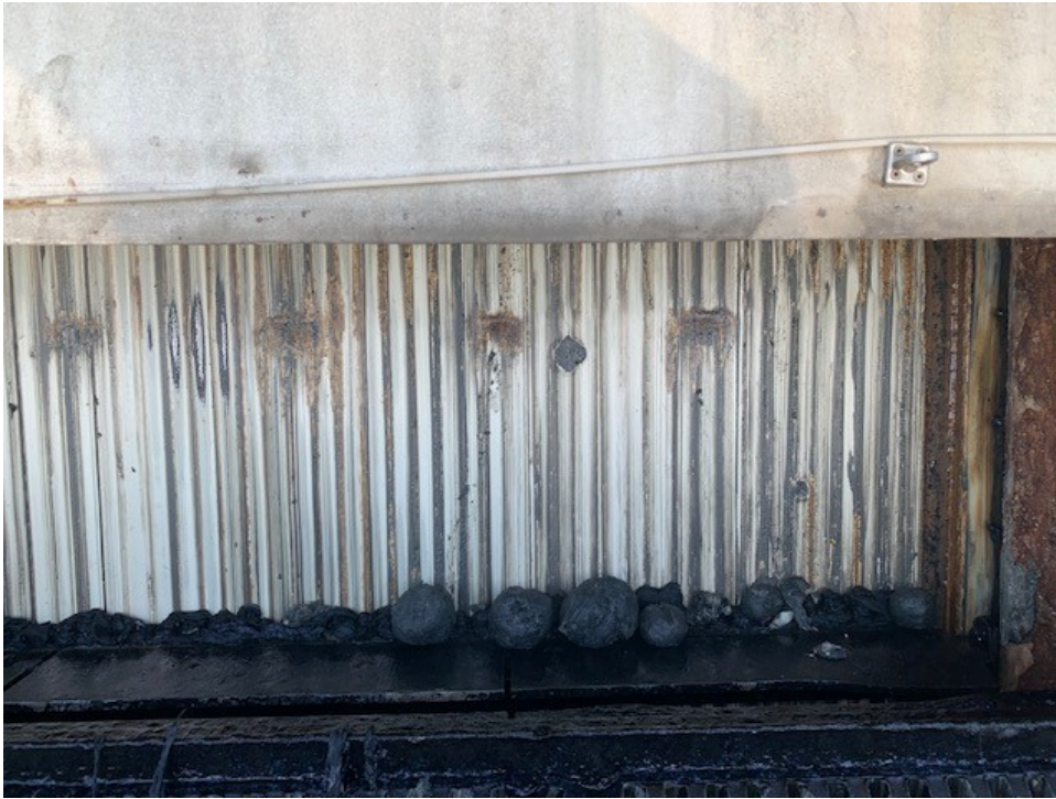
Figure 1: Bar screen #1 at JWPCP on 9-8-2021 with the observed greasy material, including grey grease balls about the size of grapefruits.
