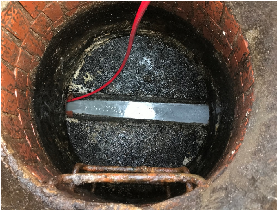
Figure 11: Local line manhole after cleaning on 3-30-2021.
