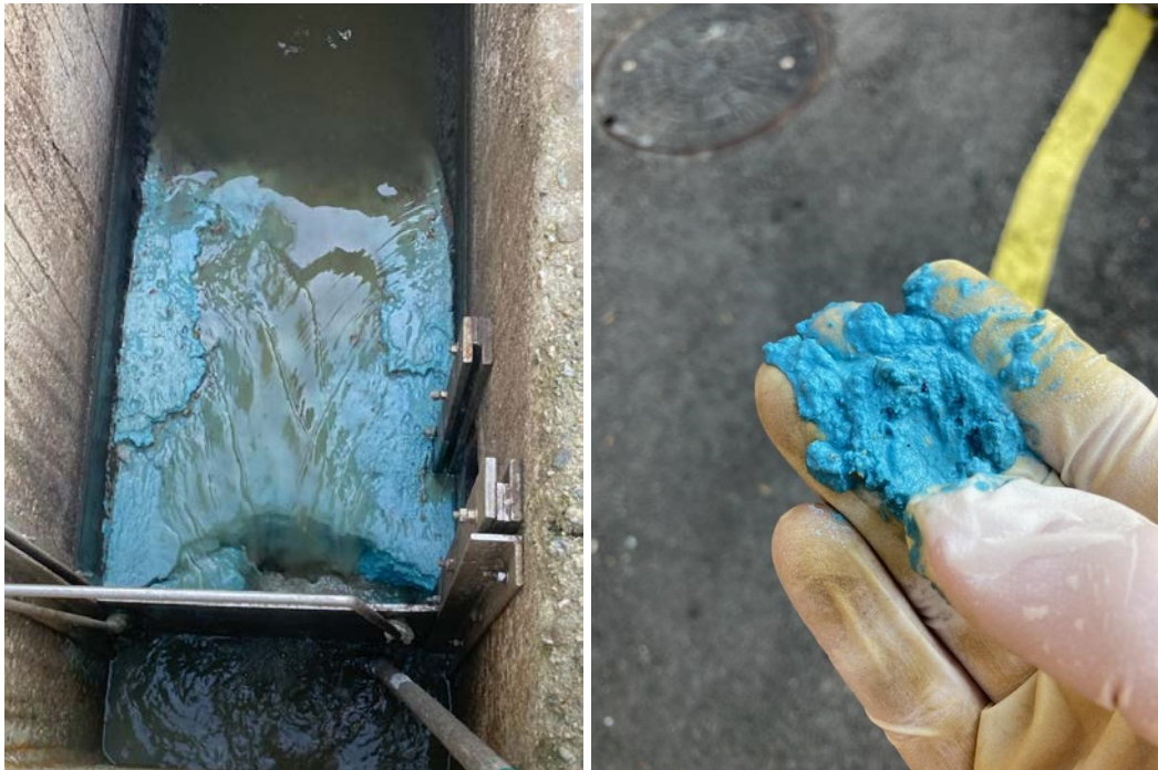
Figures 7 and 8: The blue solids present in the influent channel at the La Cañada WRP on 8-13-2021.
