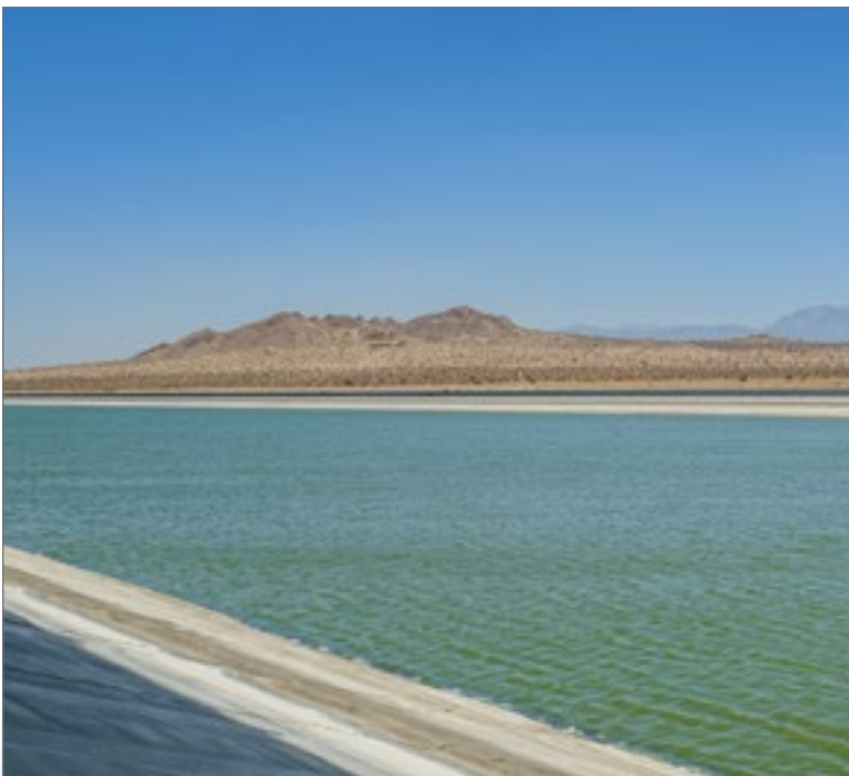
Recycled water is stored in one of the Palmdale WRP’s two reservoirs
