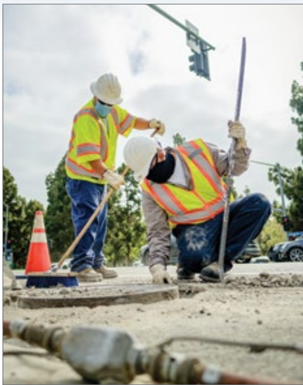
Two of our 1,700 employees performing sewer maintenance work
