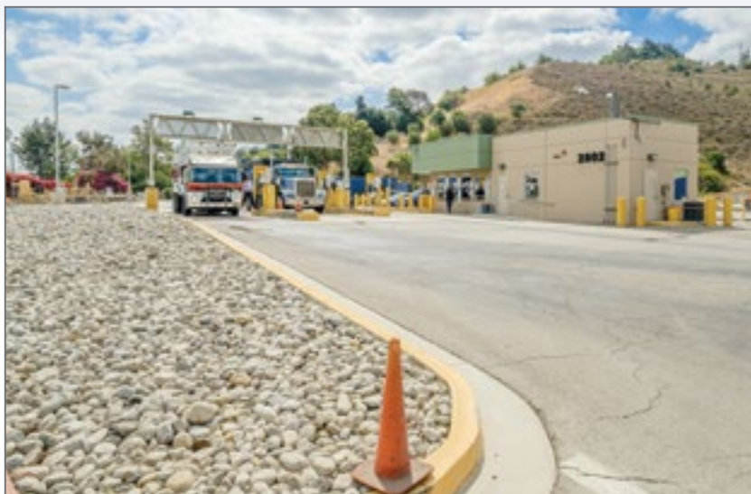
Trucks being weighed at the Puente Hills Materials Recovery Facility scales
