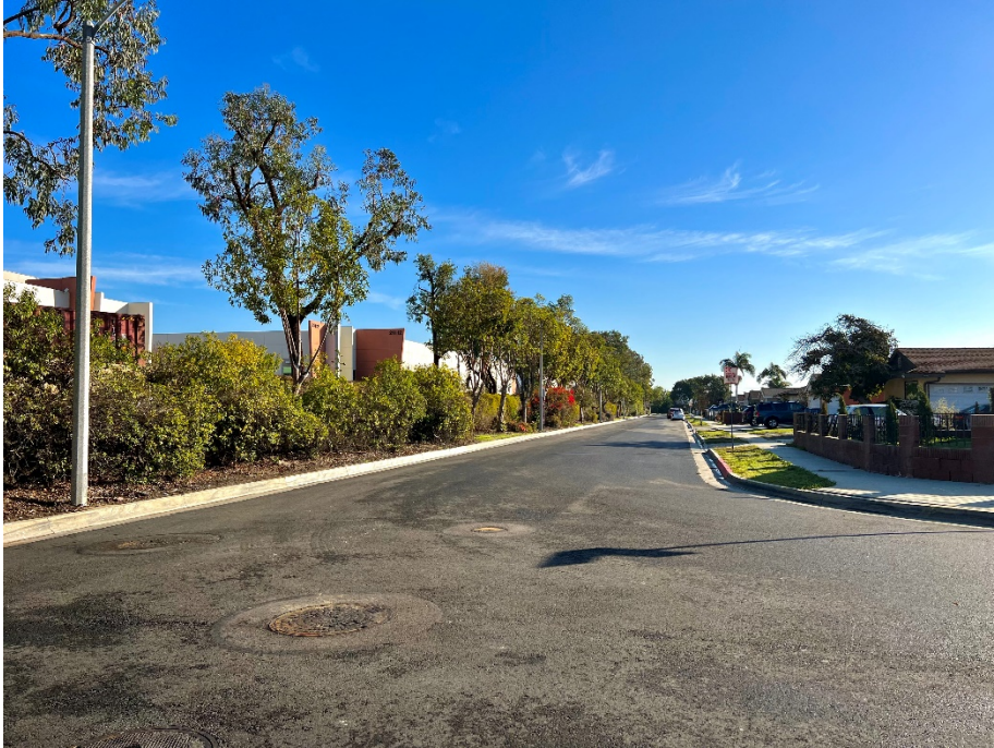
Photo 15: West 212 th Street on January 1, 2022 at 9:22 a.m. after initial cleaning of the areas affected by the SSO was completed. View facing east at intersection of West 212 th Street and South Lynton Avenue.
