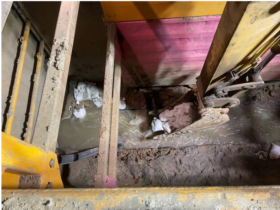
Photo 22: Wastewater flow restored to the sewer on January 3, 2022 at approximately 6:00 p.m.
