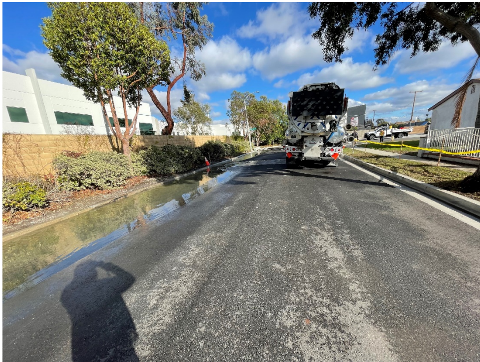
Photo 10: West 212 th Street facing east toward South Moneta Avenue on December 31 at 2:04 p.m. The overflow was significantly reduced and contained to the north gutter (at left) during the entire day due to the operation of four bypass pumps.
