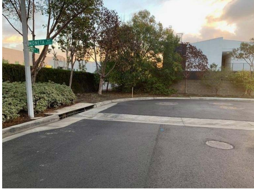
Photo 3: Catch basin where the SSO entered the storm drain system. View facing east on West 212 th Street, west of the intersection with South Moneta Avenue.
