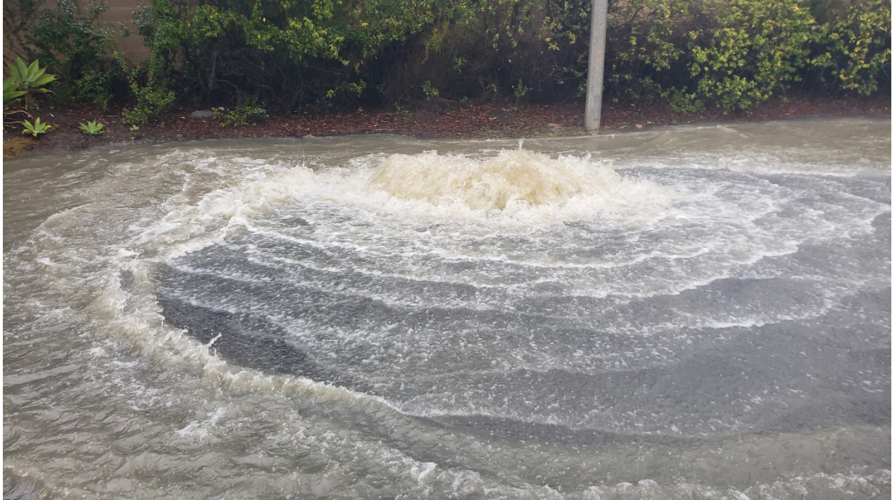
Photo 1: Wastewater overflowing from LACSD MH 08 0719 during SSO event on December 30, 2021 at 2:15 p.m. immediately after arrival of LACSD staff. View facing north at the intersection of West 212 th Street and South Lynton Avenue.
