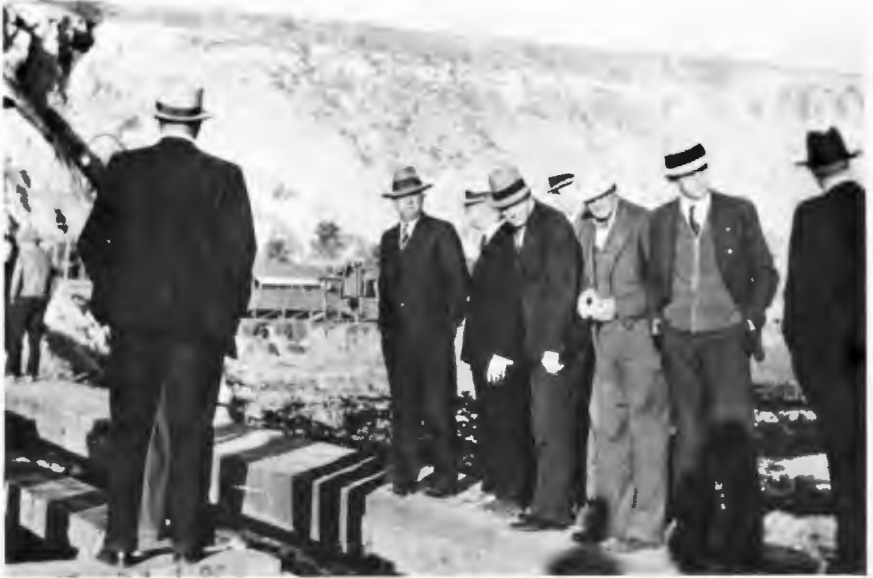
DISTRICT DIRECTORS AT WHITE'S POINT — The directors made frequent trips of inspection. This one, made on November 12, 1935, occurred during construction of the White's Point tunnel and ocean outfall.
