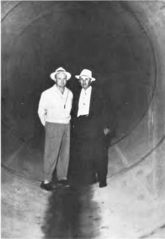
INTERIOR OF TWELVE-FOOT DIAMETER REINFORCED CONCRETE PIPE—A joint outfall trunk sewer built in 1955. Contractor Vido Artukovich, on right; John Parkhurst, Engineer, C.S.D. (later Chief Engineer and General Manager of C.S.D.).
