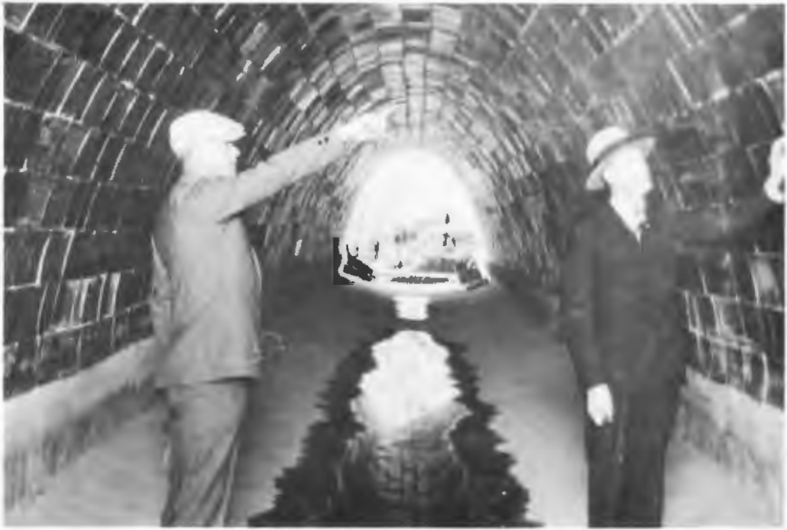
TILE-LINED CONDUIT — Typical conduit section: 10' 6" reinforced concrete, basket section, vitrified clay liner plates in sides and crown. Looking toward entrance to joint disposal plant. December, 1927. Rawn (left), newspaper representative (right).
