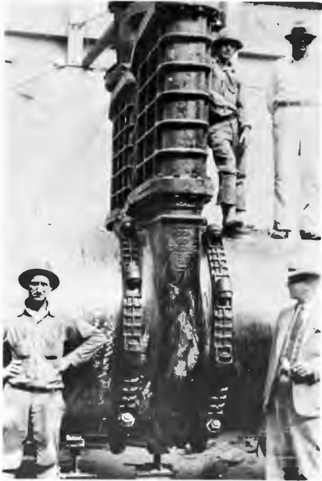
GATE VALVES—TUNNEL TO OCEAN OUTFALL —Sixty-inch diameter gate valves were placed at the shore ends of the two ocean submarine pipes at White's Point. They have been in frequent use in revision and extension of the lines.
