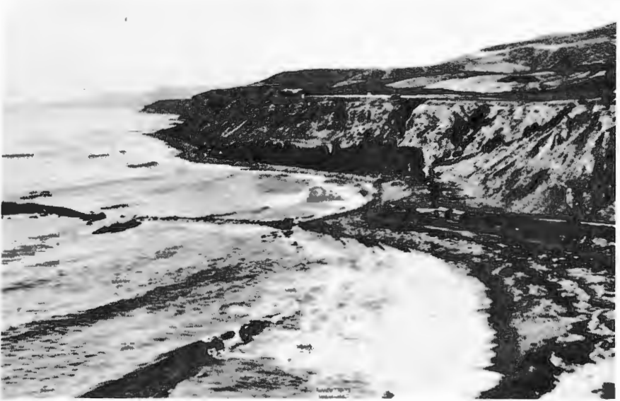
WHITE'S POINT — The tunnel emerged from the right at inert elev. -12 ft., U.S.G.S. datum. The ocean outfall extended seaward (to the left), following along the near side of the reef (center of picture).
