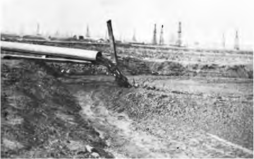
DIGESTED SLUDGE PUMPED TO SHALLOW LAGOONS —Liquid sludge delivered to shallow lagoons contained some 95% liquid. A large part of this separated from the sludge and drained away. The rest was removed through evaporation.
