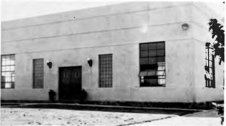
SEWAGE PUMPING STATION—Long Beach Main Pumping Station, District 3. Current capacity about 35 M.G.D.
