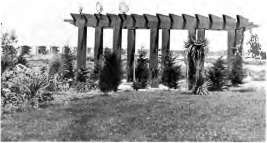
HOLLYWOOD-RIVIERA PUMP STATION —Because of its surroundings the Hollywood-Riviera Pump Plant was all placed below ground and disguised on the surface with a pergola. Some of the posts served as vents for the pump room.
