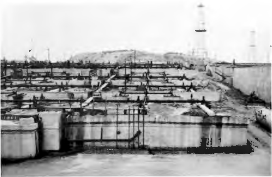
EARLY MULTISTAGE TANKS —First of the multistage digestion tanks at Bixby. These tanks were later supplemented by other similar tanks; and still later (1960 or so) were discontinued in operation in favor of others of greater efficiency.
