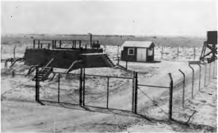
PRIMARY PLANT AT LANCASTER — First plant at Lancaster, District 14. Imhoff tank. Disposal of effluent to neighboring slough area.
