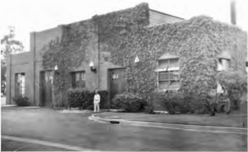
BIXBY POWER PLANT —The first Chief Engineer's preference for brick construction is demonstrated in the original power plant at Bixby. Built in 1936, the building was converted to concrete exterior finish later to bring it into harmony with other structures.
