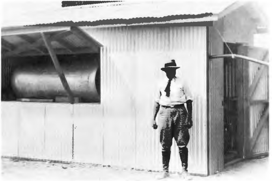
PORTABLE ONE-TON CHLORINATION STATION, 1931 — Chlorination stations were constructed (1931) so as to be easily moved from one location to another. All stations were designed for one-ton containers. Fred Bowlus, Construction Engineer, in picture.
