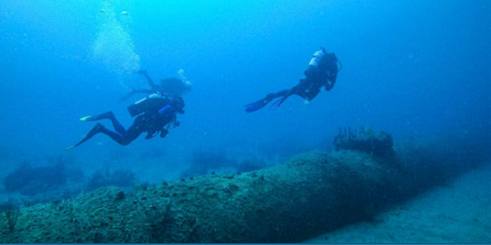
Divers inspect an ocean outfall pipe.
