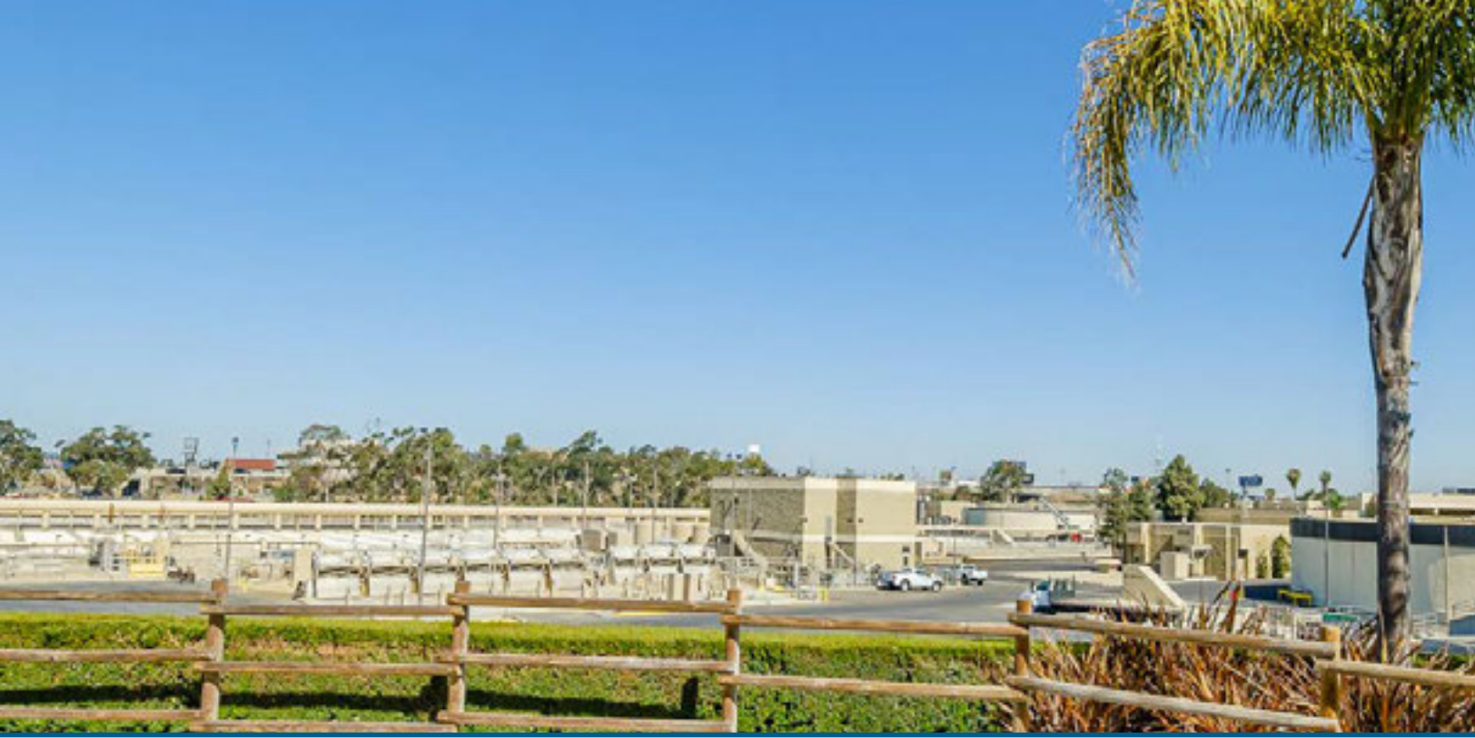
Overlooking primary treatment at the Warren Facility.
