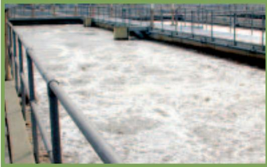
Bacteria and other microorganisms are the “good guys” in the wastewater treatment process, where they help clean wastewater by feeding on the organic material in it. In the aeration tanks to the left, the microorganisms, not the waste, make the water brown. Air is bubbled through the tanks so the microorganisms can breathe.
