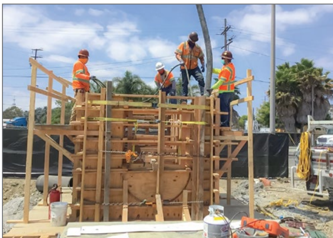
Diversion structure construction at Carriage Crest Park.
