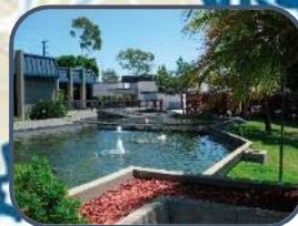
City of LA Terminal Island Water Reclamation Plant
