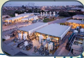
West Basin MWD Edward C. Little Water Recycling Facility
