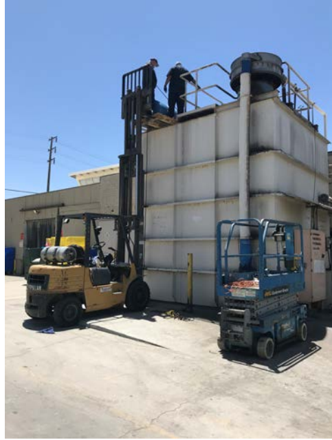
Figures 5 and 6: Pink colored wastewater in the flume at Mission Linen Supply and the company personnel manually adding bleach into the facility's above-ground flow equalization tank to remove the color prior to discharge.
