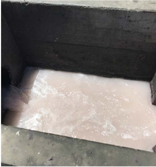
Figures 5 and 6: Pink colored wastewater in the flume at Mission Linen Supply and the company personnel manually adding bleach into the facility's above-ground flow equalization tank to remove the color prior to discharge.
