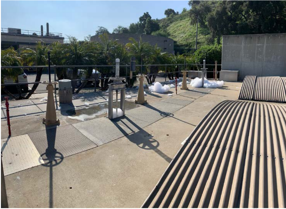
Figure 6: Picture of heavy white foam in primary channel #1 at the Pomona WRP at 0900 hours on 4-14-2020.
