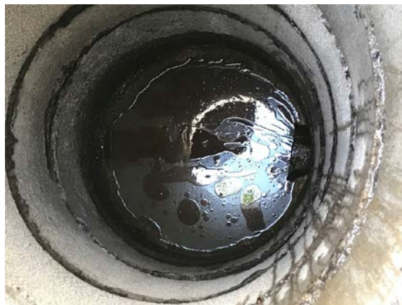
Figures 3 and 4: 12-17-2020 photos showing the stuffed chicken fryer that caught fire and oil residual floating on the top of the wastewater in the industrial wastewater sampling box at Signature Fresh. Note also the oil on the floor next to the fryer.
