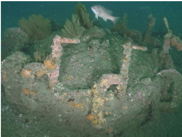
Figure 62: Six C-clamps were installed onto the inner most raised manhole in late 2015 on the 60-inch outfall.
