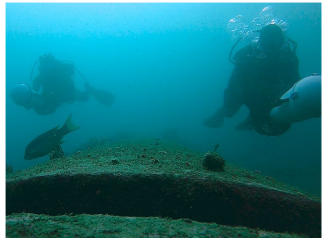
Figure 21: Divers inspecting an outfall.
