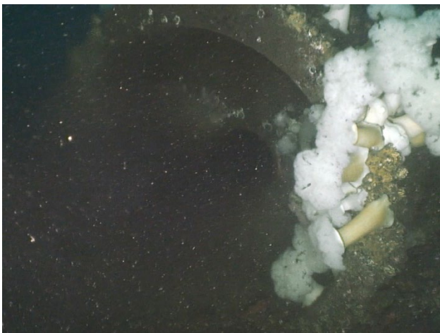
Figure 39: Terminus port with flow on the east diffuser leg of the 90-inch outfall.
