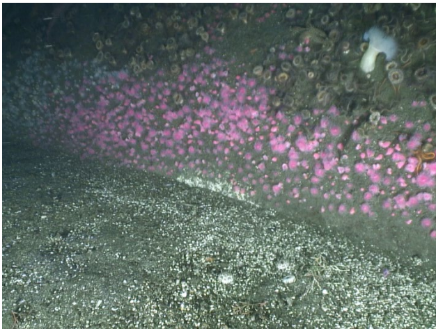
Figure 22: A buried port with no flow, 10 th from the terminus, on the north side of the 120-inch outfall.
