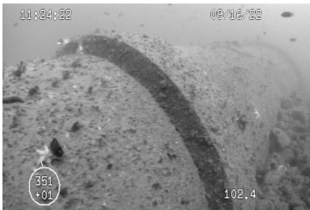
Figure 3: A concrete bell and spigot joint on the 120-inch outfall.
