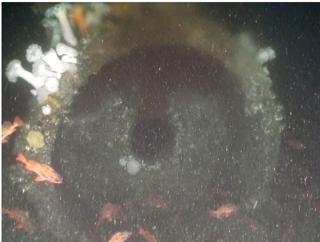
Figure 38: Terminus port with flow on the west diffuser leg of the 90-inch outfall.
