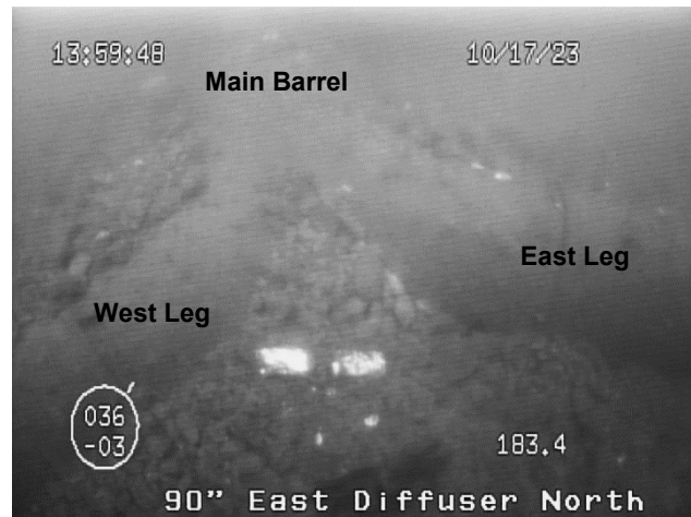
Figure 36: Wye structure on the 90-inch outfall.
