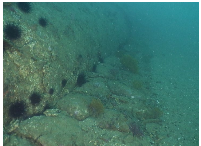
Figure 61: Sand/cement bags placed along the 60-inch outfall during the 1997 reballasting project.
