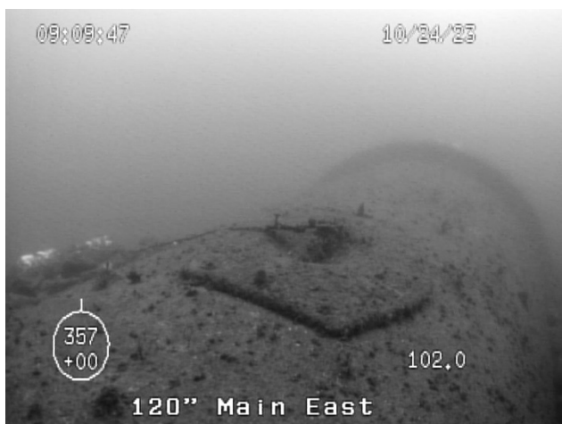
Figure 34: Attached anode on the 120-inch outfall.
