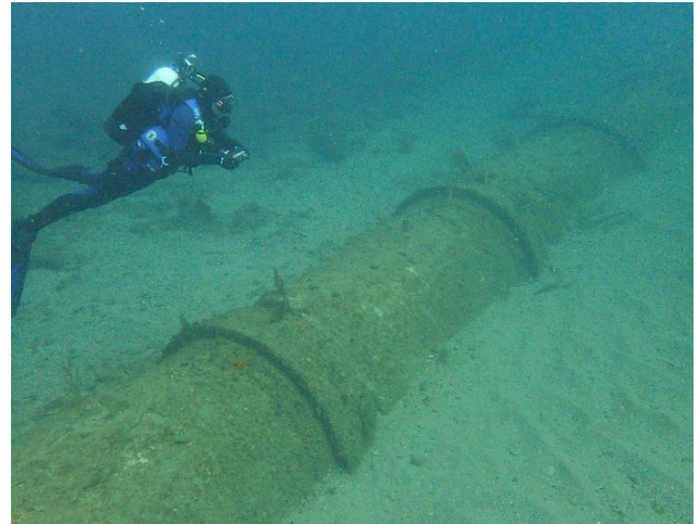
Figure 16: Cast iron joints on the 60-inch outfall.
