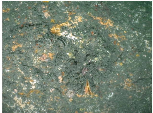
Figure 60: Barnacle collar formed around and over a port on the 60-inch outfall.
