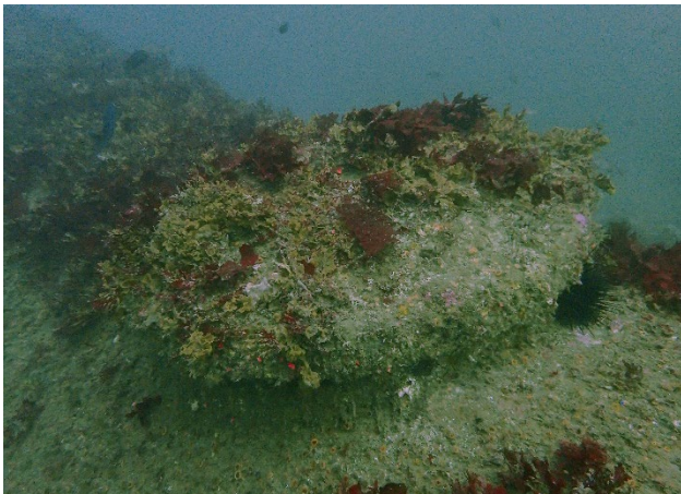
Figure 15: A raised manhole cover on the 72-inch outfall. This type of manhole cover is also on the 60-inch outfall.
