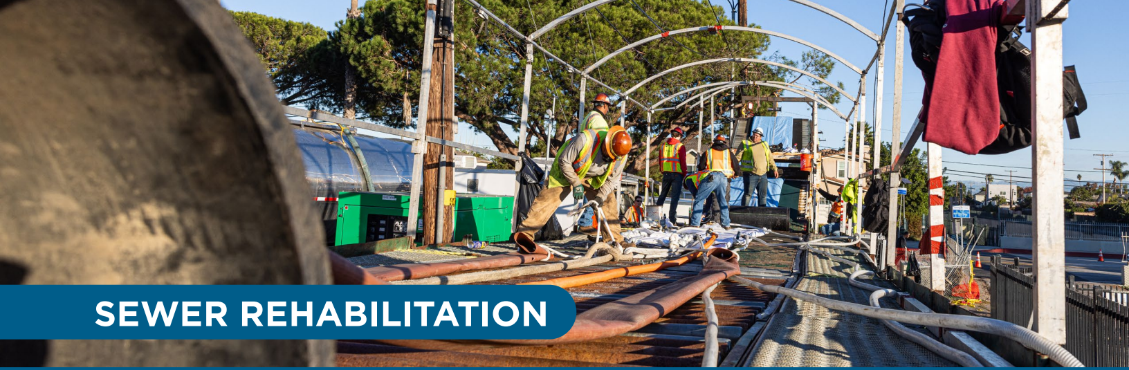
Crews rehabilitating an aging sewer in Gardena using cure-in-place-pipe method
