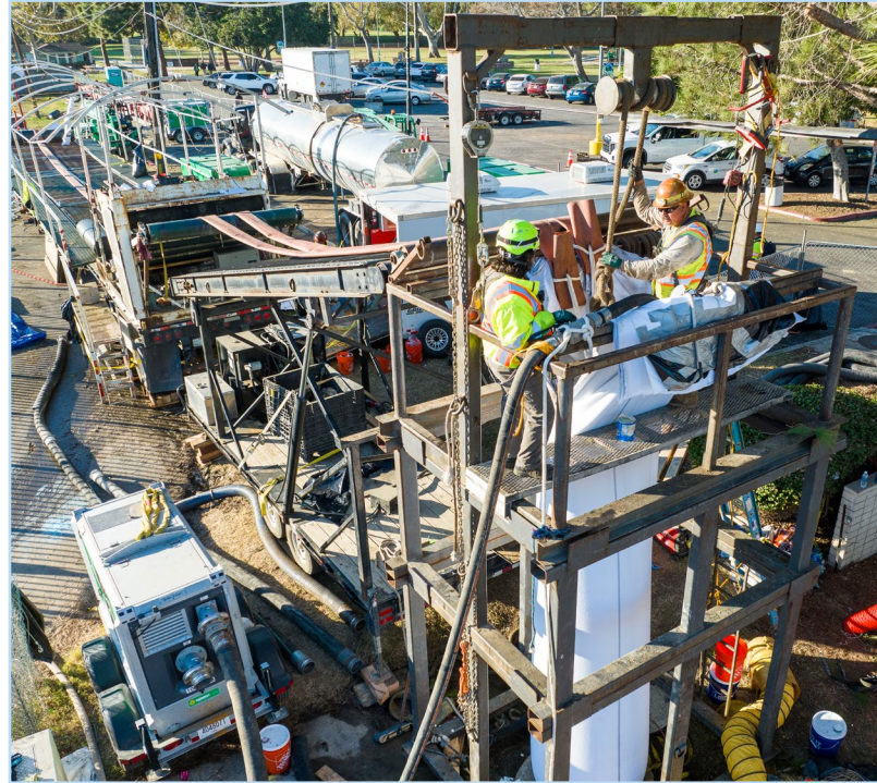
ABOVE FROM LEFT: The Clearwater Tunnel ; a sewer rehabilitation project in Gardena using the CIPP method BELOW FROM LEFT: Sewer rehabilitation work in Carson ; the renaming of the Pure Water Southern California Demo Facility in honor of Congresswoman Grace F. Napolitano
