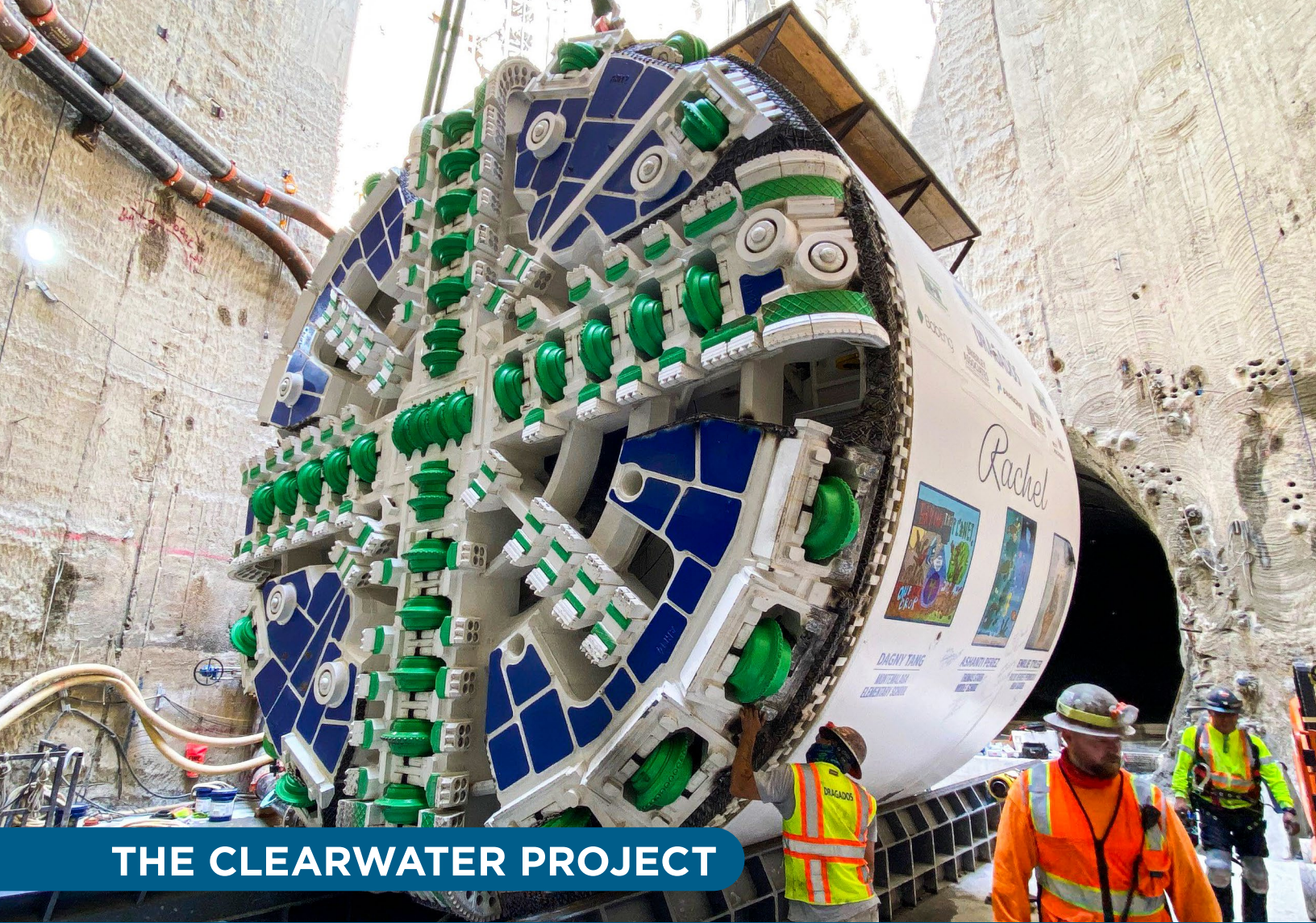
ABOVE: The tunnel boring machine, Rachel, being assembled
