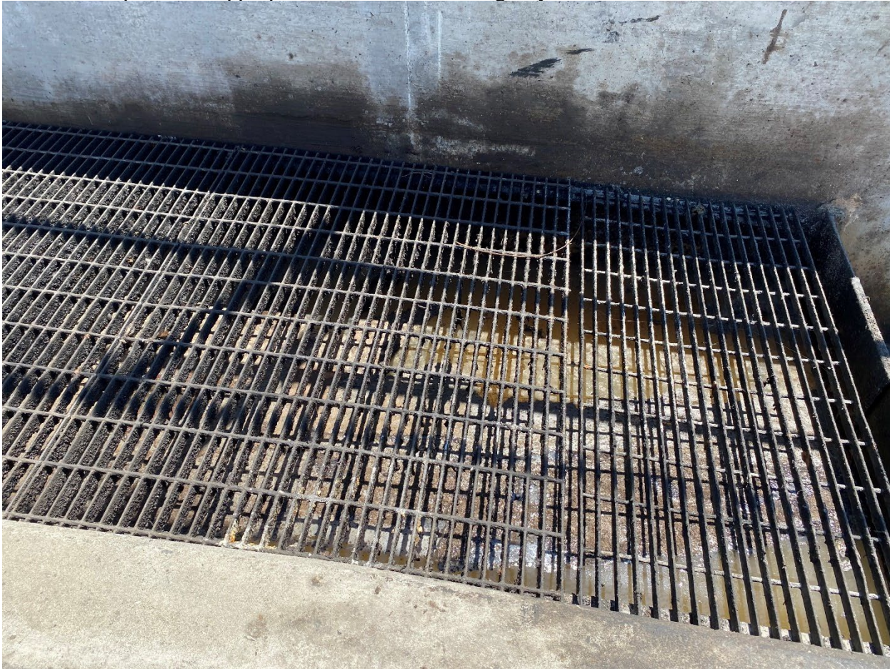
Figure 17. Trench Prior to Storm Drain
