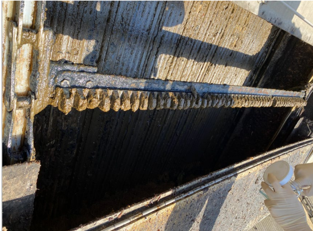
Figure 19. Food waste collected on the J.O. "A" inlet bar rakes.
