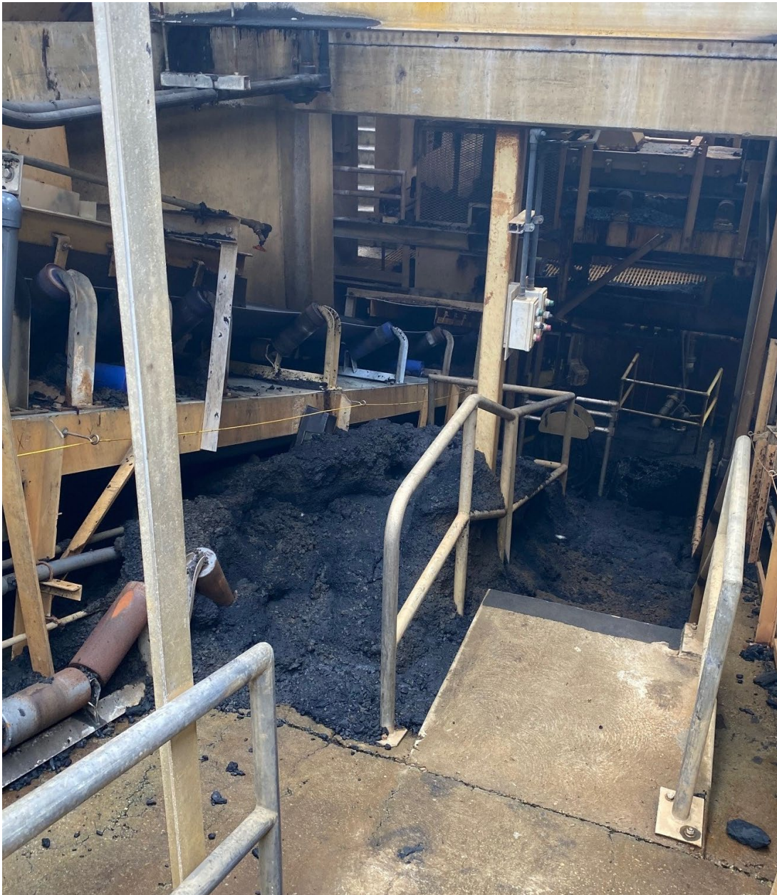
Figure 4: Excess biosolids in conveyor/sump
