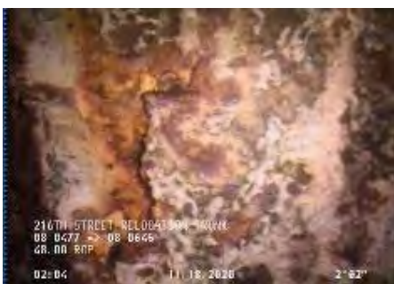
Photo 6-1 216 th Street CCTV View
