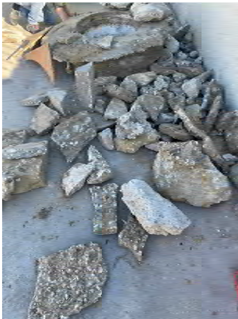
Photo 3-8 Pile of Debris from Collapse Site
