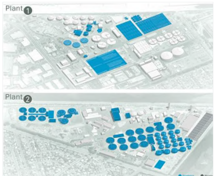
Aerial overview of OC San Plants 1 & 2.
