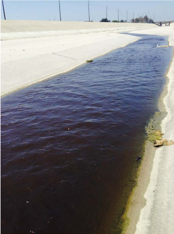
Figure 7: 5-30-14 photo of Coyote Creek looking south about a 0.8 mile upstream of the Long Beach WRP's outfall into the creek. Note the dark color of the water in the creek.
