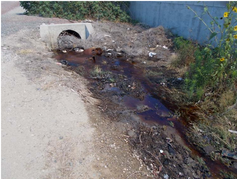
Figure 6: Storm water runoff channel downstream from the Pan Pacific Fiber facility on 5-30-14. Note the red brown color water due to the fire at the facility.
