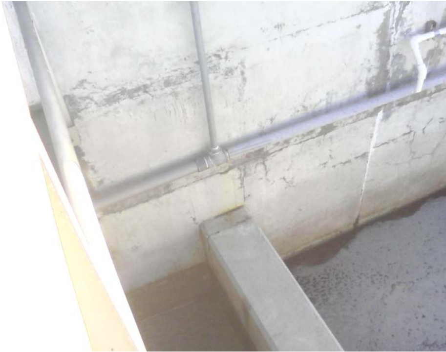
Figure 3: 12-4-14 photo of pink colored staining on a filter tank wall at Whittier Narrows WRP.
