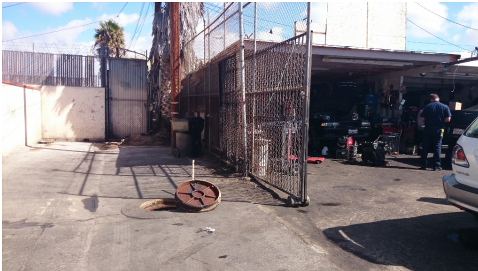
Figure 1: Photo taken on 4-1-14 showing local line sewer manhole located in the alley behind 10101 Hawthorne Blvd in Inglewood. Note the palm tree directly behind the manhole where some waste used oil was noted that had appeared to have been dumped onto the tree roots.
