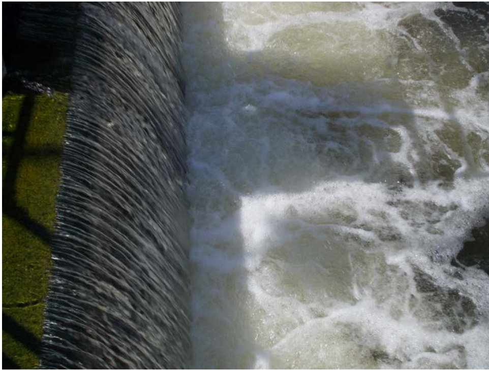
Figure 4: LCWRP outfall photo taken at 1230 hours on 10-9-14. No color present.
