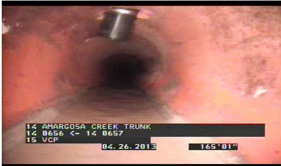
Figure 5: 4-26-13 CCTV screen grab showing the illegal 4" line connection on the 15" Amargosa Creek trunk sewer in Lancaster.
