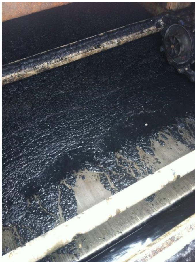
Figure 5: E-3 south battery primary skimmer black solids observed on 7-30-15. Note how the solids appear essentially visually identical to that of a black oily material.
