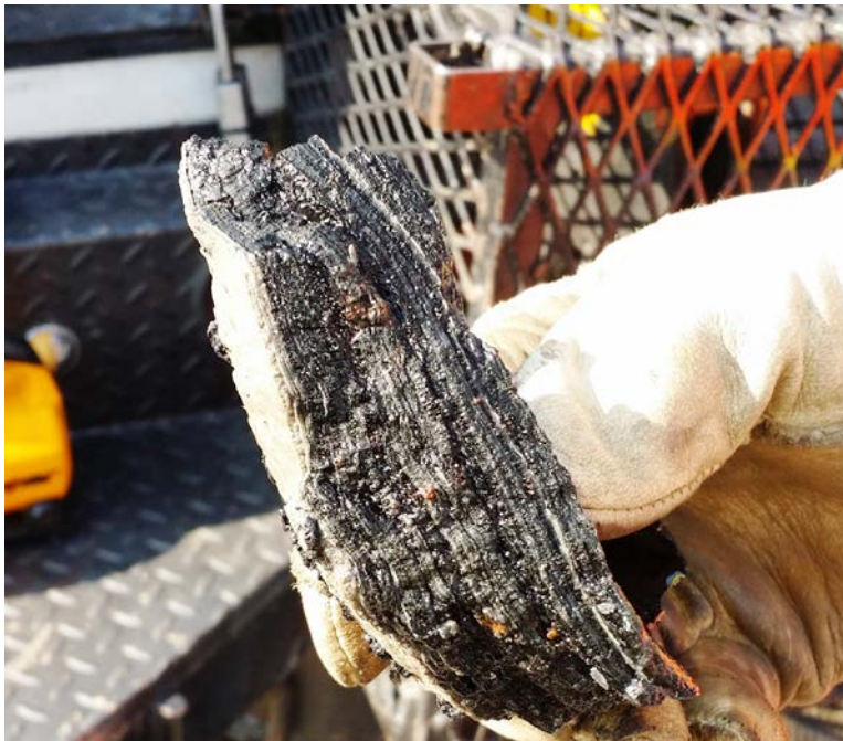
Figure 8: Piece of the scale removed from MH 2214A on 4-13-15. Note the layered appearance indicating it likely built up over a period of time.
