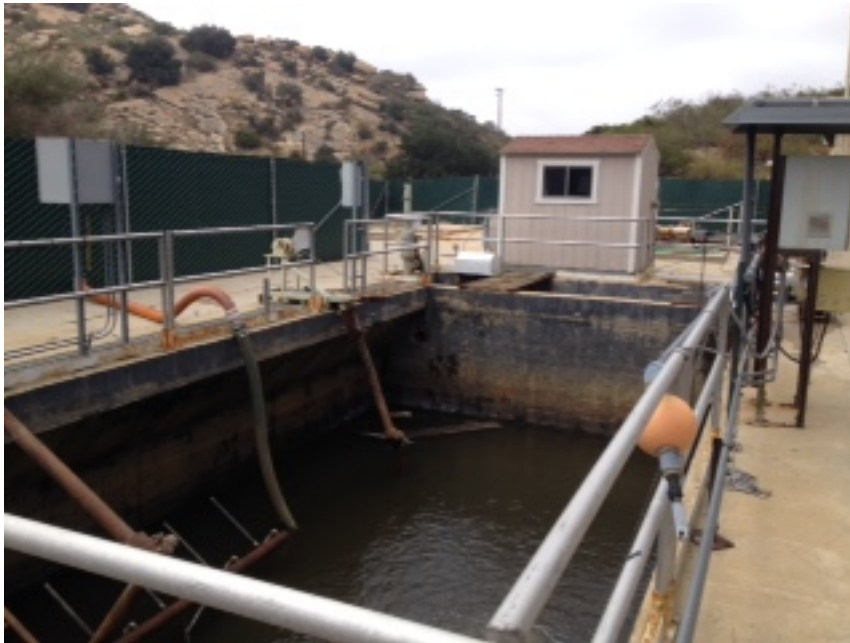
Figure 1: 5-27-15 photo of the old pocket wastewater treatment plant at the Santa Susana facility that now functions as a septic waste collection tank.
