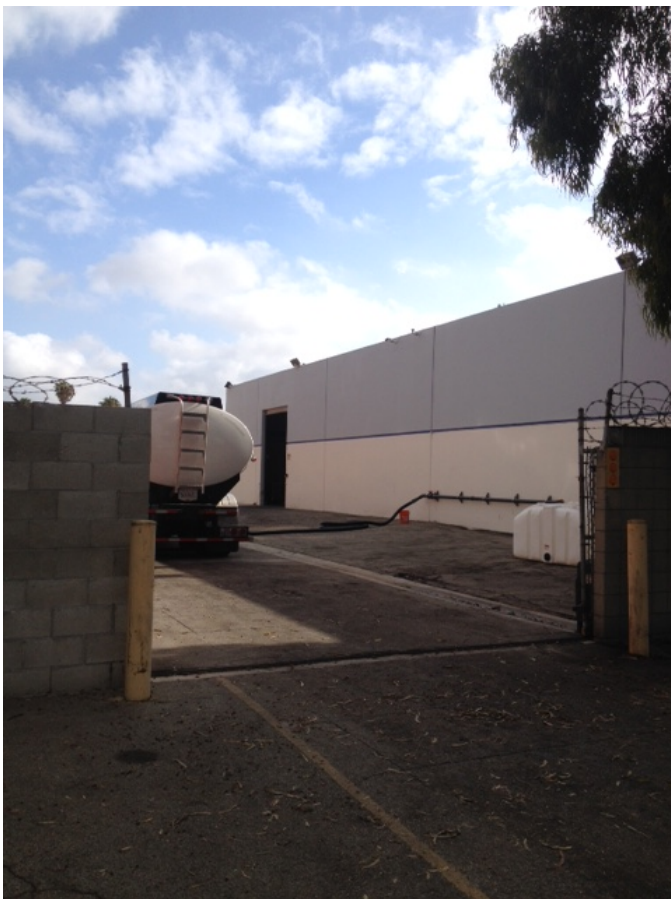
Figure 1: 7-9-15 photo of tanker truck loading/unloading Area at SPF Terminals in Compton. Note the white tote used for wastewater storage against the building and adjacent storm water swale which was found to have small amounts of alkaline (pH=9) water.
