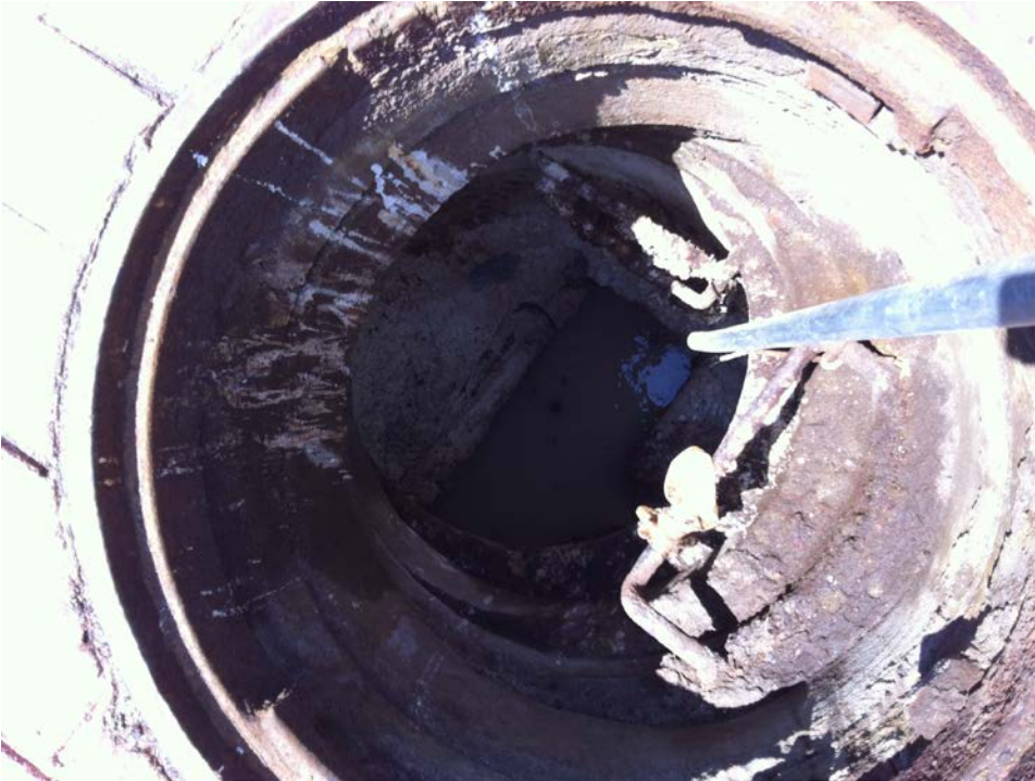
Figure 3: 5-20-15 photo of MH 18 1083.
