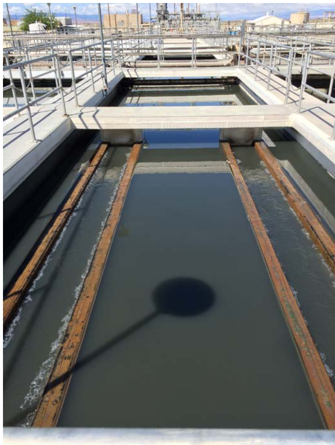
Figure 2: 4-8-15 photo of a primary tank at Lancaster WRP. Note the dark color present.
