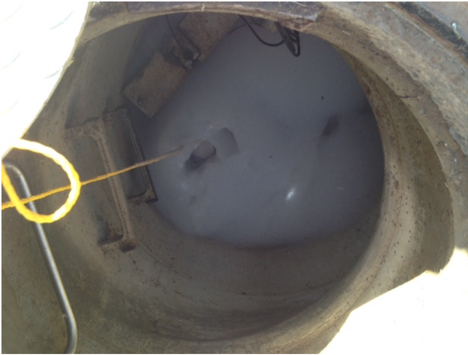
Figure 9: Several feet of white foam noted above the industrial wastewater monitoring flume at Northrup Grumman Site 3 permit location #14934 at 1230 hours on 11-17-15.
