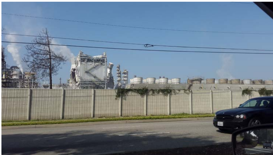
Figure 4: Inspector street view photo looking west from Crenshaw Boulevard at the ESP unit on 2-18-15. Note the walls of the unit have been bowed and blown outward by the force of the explosion in the unit.
