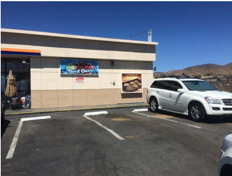
Figure 6: 1500 gallon septic tank system located in the parking lot of the Arco AM/PM facility on 9-17-15.
