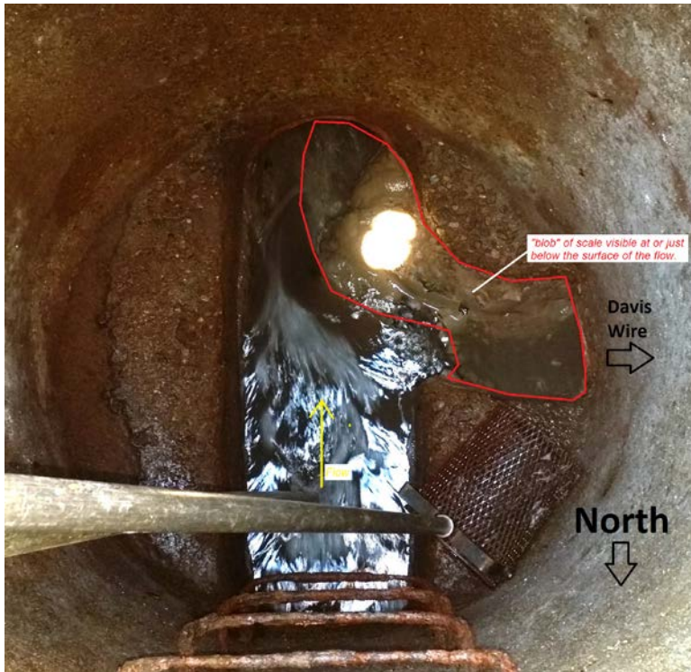
Figure 7: White or grey scale in MH 22 1214A on 4-13-15.
