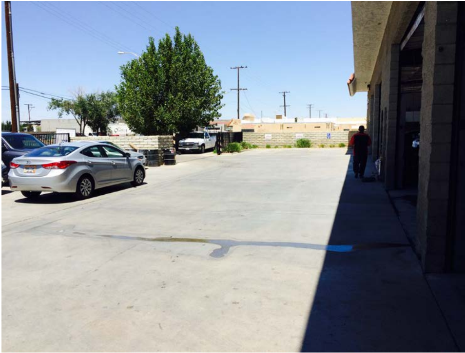
Figure 3: Minor amount of wastewater in front of Precision Auto Body Repair observed by I.W. Inspector Jonathon Powell on 7-28-15.
