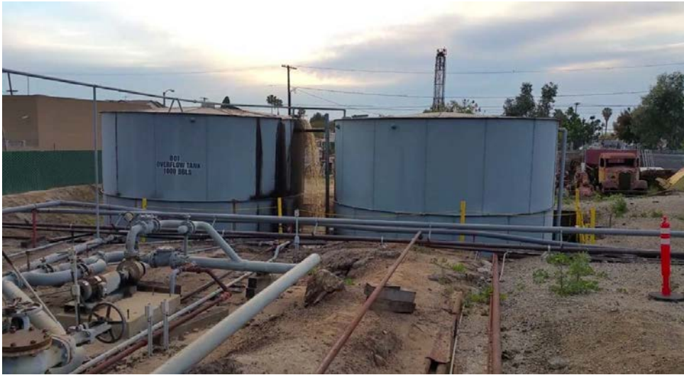
Figure 1: Photo taken at 1830 hours on 3-17-15 of the ongoing spill of oily wastewater from the “001 OVERFLOW TANK” at the Oil Operators facility in Signal Hill.
