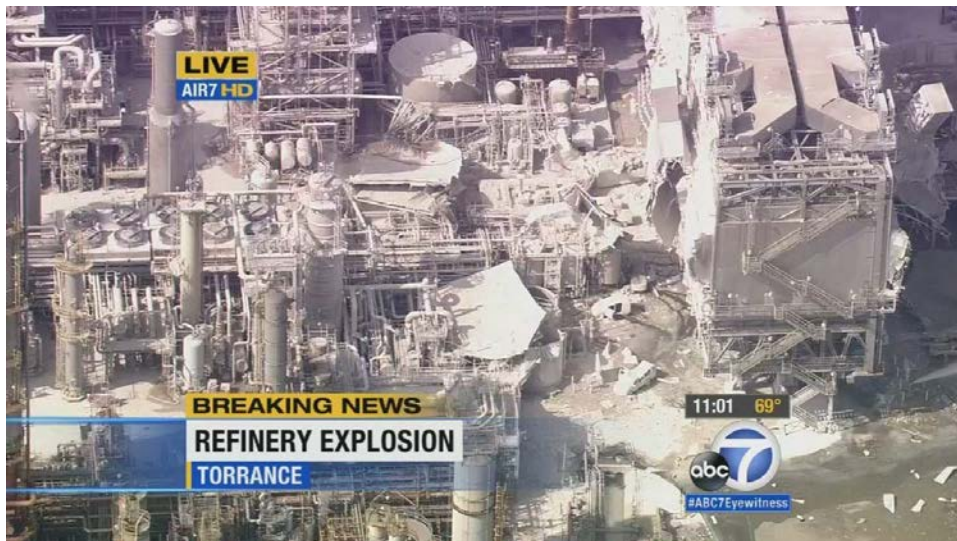
Figure 5: KABC News helicopter picture of the damaged ESP unit and surrounding area covered in debris.
