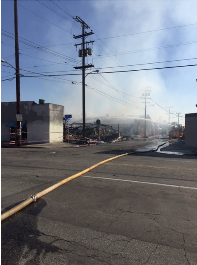
Figure 8: Photo taken by Senior I.W. Inspector Bill Barnum upon arrival at the scene of the 10-7-15 fire that occurred in an unincorporated area of Los Angeles County west of the city Huntington Park known as “Florence.”
