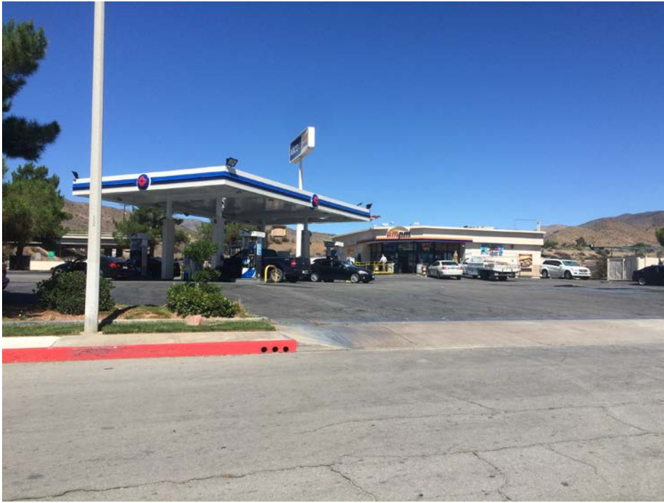
Figure 5: Arco AM/PM located at 33488 Crown Valley Road in Acton on 9-17-15.
