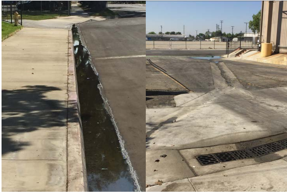
Figures 4 and 5: Spilled process wastewater noted at Partners Alliance Cold Storage on 8-27-15.
