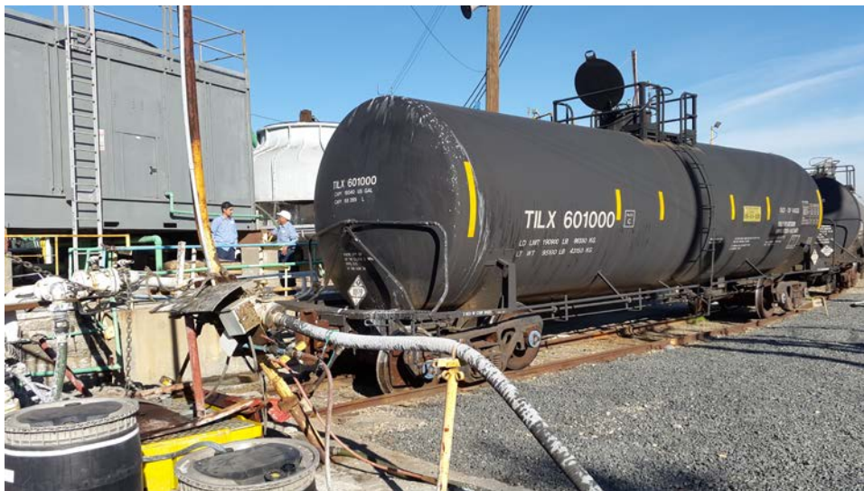
Figure 5: 1-16-15 photo taken by Inspector Placencia showing the railroad tanker car that overran its normal stopping point where it smashed into a 3" caustic transfer line and potable water pipe.
