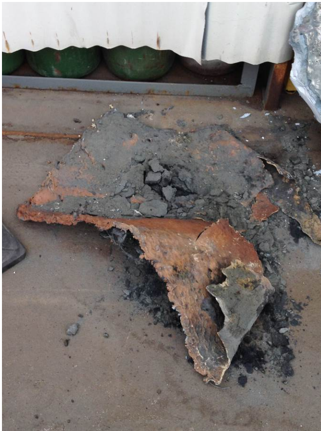
Figure 12: Photo of liner material, epoxy resin and dark solids removed from Manhole 03 0427 on the Water Street trunk on 4-16-15. Note the orange color of the liner that matches that in Figure 11 above.
