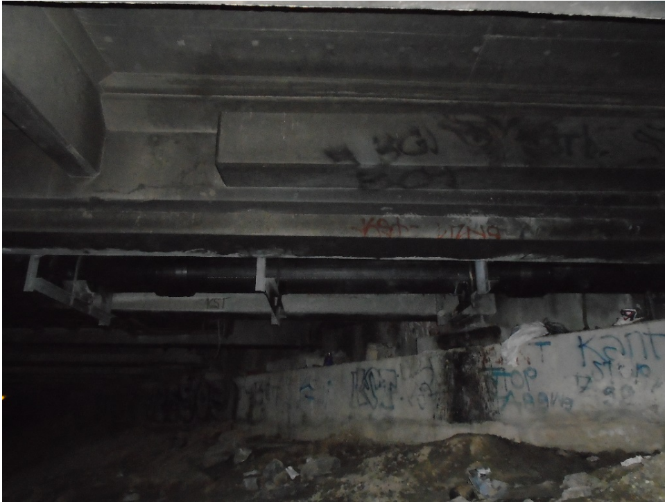
Figure 7: The 14" WBMWD brine line following completion of repairs.
