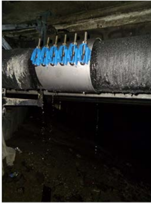
Figures 2 and 3: 1-14-16 temporary repair sleeve installed on the damaged 14" brine line.
