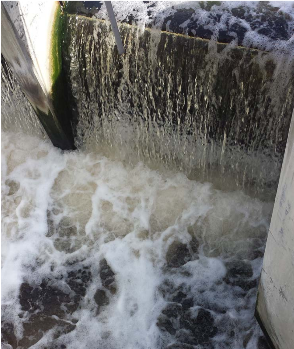
Figure 2: Los Coyotes final effluent on 2-18-16 at 1117 hours. Note slight brown tint in the forebay waters.
