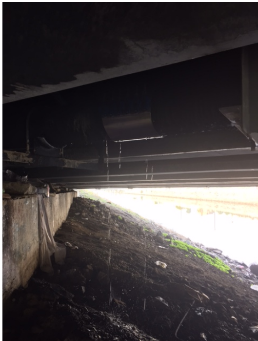
Figures 2 and 3: 1-14-16 temporary repair sleeve installed on the damaged 14" brine line.
