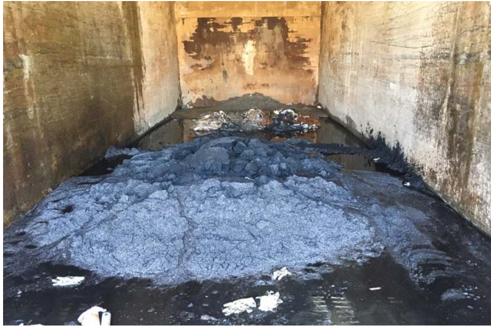
Figure 12: Sand removed from the local sewer by DPW and brought to JWPCP for disposal.
