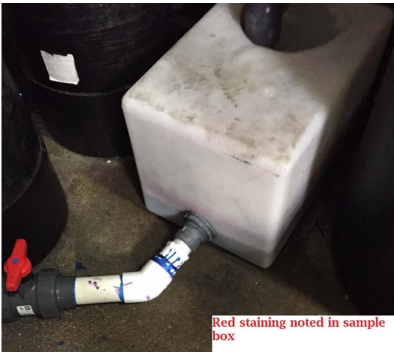
Figure 11: Pink staining present in the OCCS sample box on 6-16-16.
