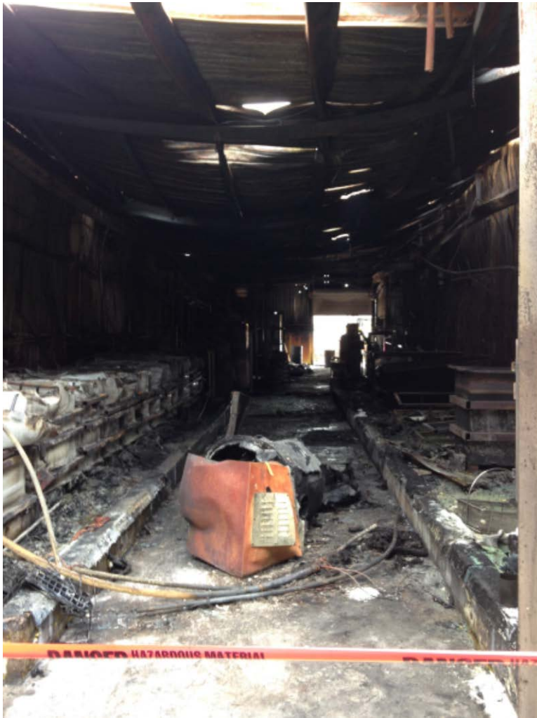
Figure 4: Photo showing the fire damaged metal processing area at Bodycote Thermal Processing on 9-4-16. Note the partially melted open-top white poly plating tanks on the left.
