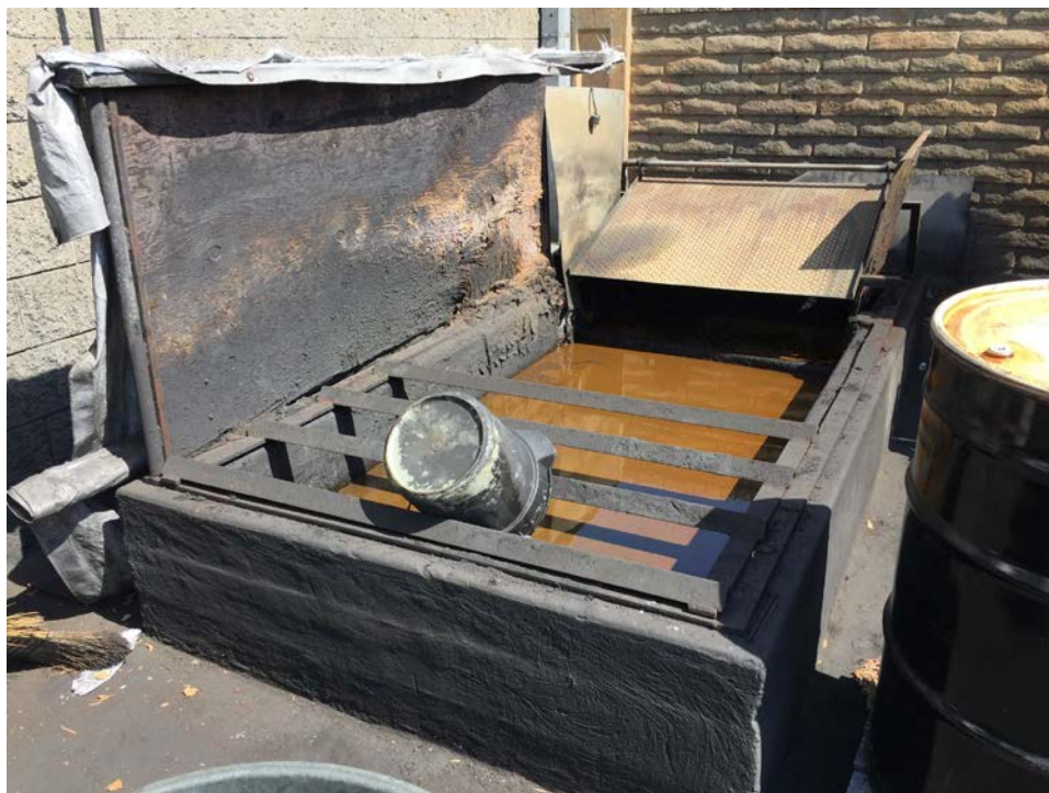
Figure 8: Waste water-based coolant evaporation pit at Carbro Corp.
