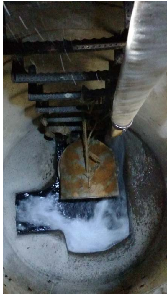
Figures 5 and 6: “Blow off” connection where a 3” diameter firehose is being used to tap into the water in the underground brine line and the same firehose line as it discharges into the local discharge line manhole. Note the absence of any surcharging.
