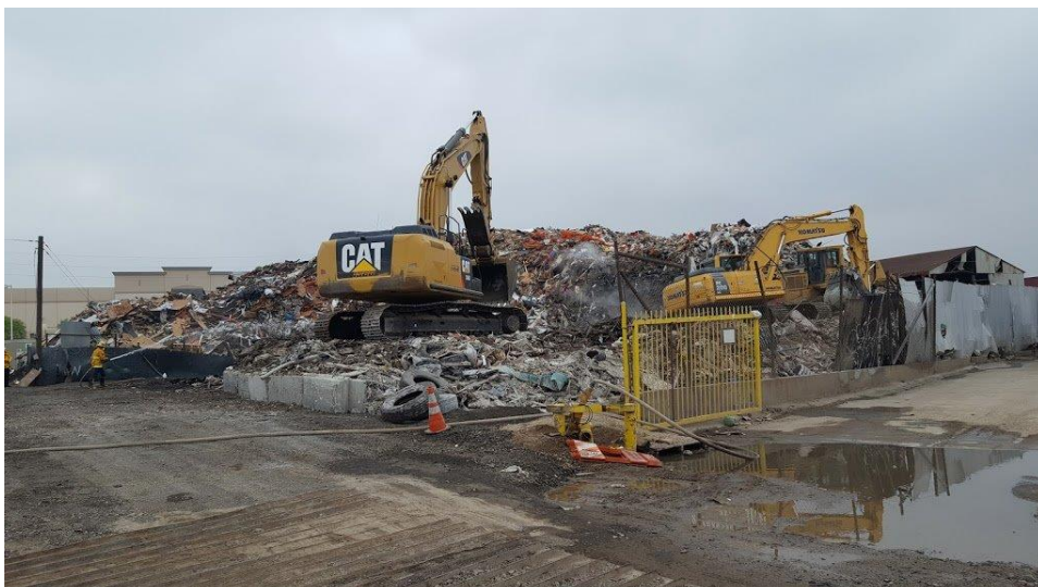
Figure 3: 10-11-16 photo of debris/waste pile being slowly removed by excavators.
