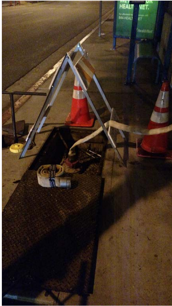
Figures 5 and 6: “Blow off” connection where a 3” diameter firehose is being used to tap into the water in the underground brine line and the same firehose line as it discharges into the local discharge line manhole. Note the absence of any surcharging.
