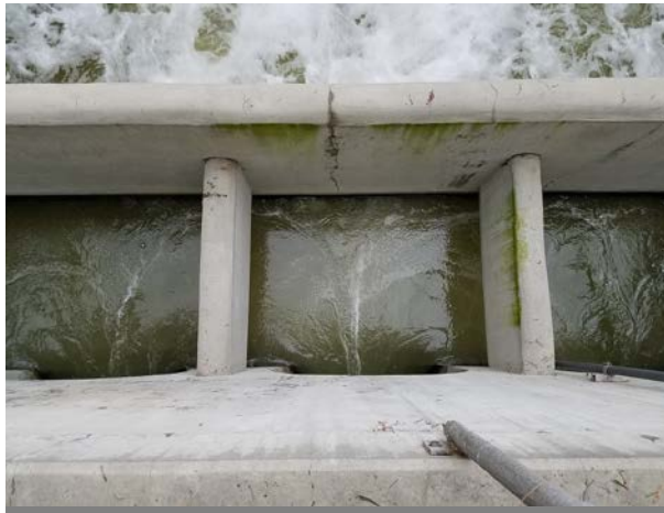
Figure 1: April 8, 2016, 6:38 p.m. photo of LCWRP forebay (top) and final effluent channel (bottom). Note the foam in the forebay but its near absence in the channel.
