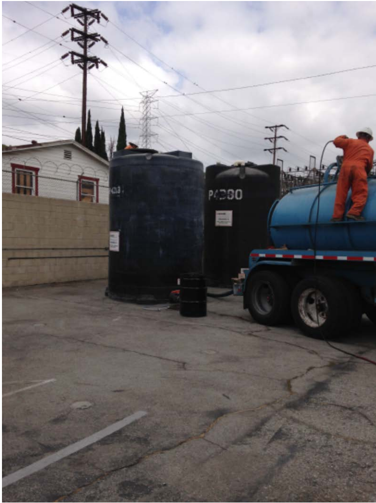
Figure 5: Portable 4000-gallon Baker tanks on-site at Bodycote Thermal Processing on 9-4-16.
