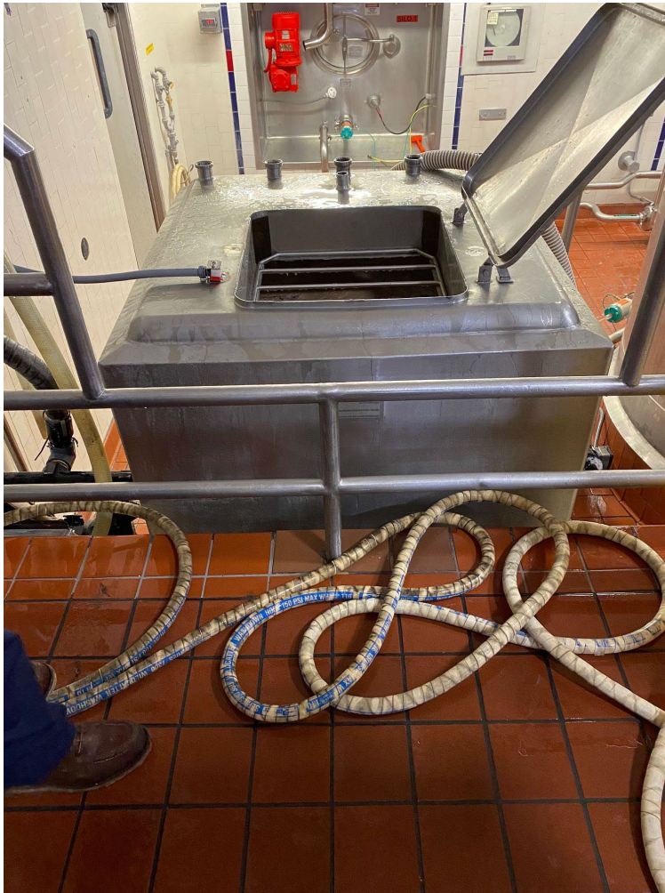
Figure 2: The 10,000-gallon capacity high BOD waste tank at Thrifty Ice Cream which is referred to by company employees as the “pig tank”.
