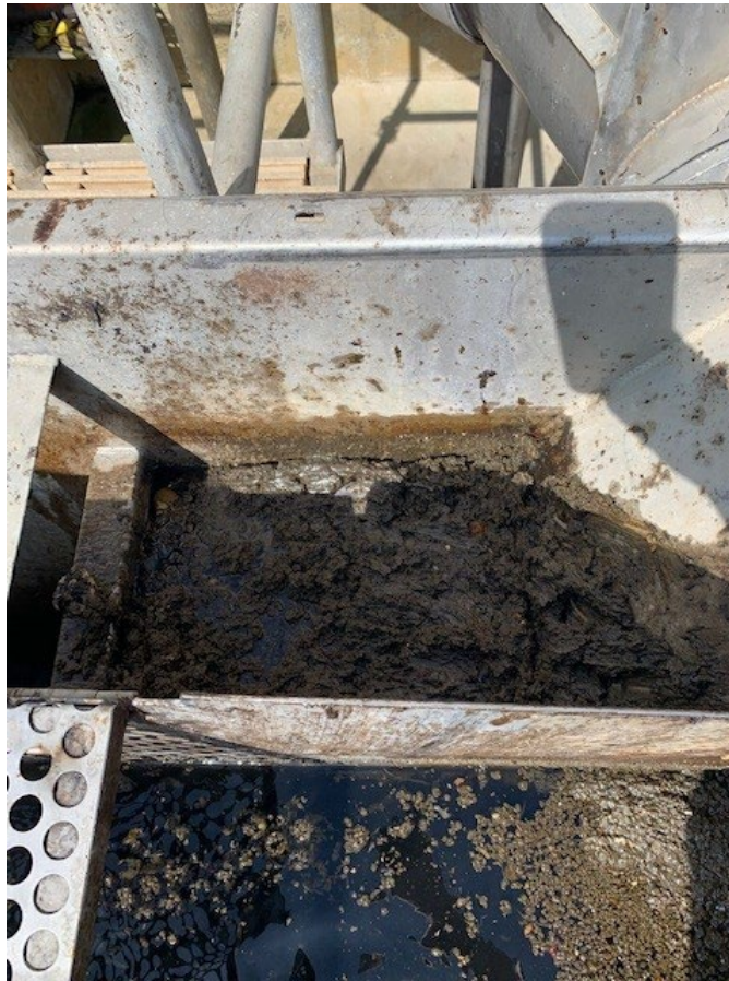
Figure 5: JWPCP North Screw Compacter 2 on August 26, 2022. Note the unusual gritty consistency of the material.
