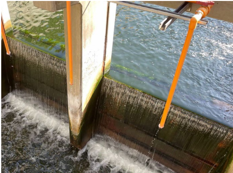
Figure 3: 3-15-22, 0800 hours LCWRP final effluent forebay. Note the green color.
