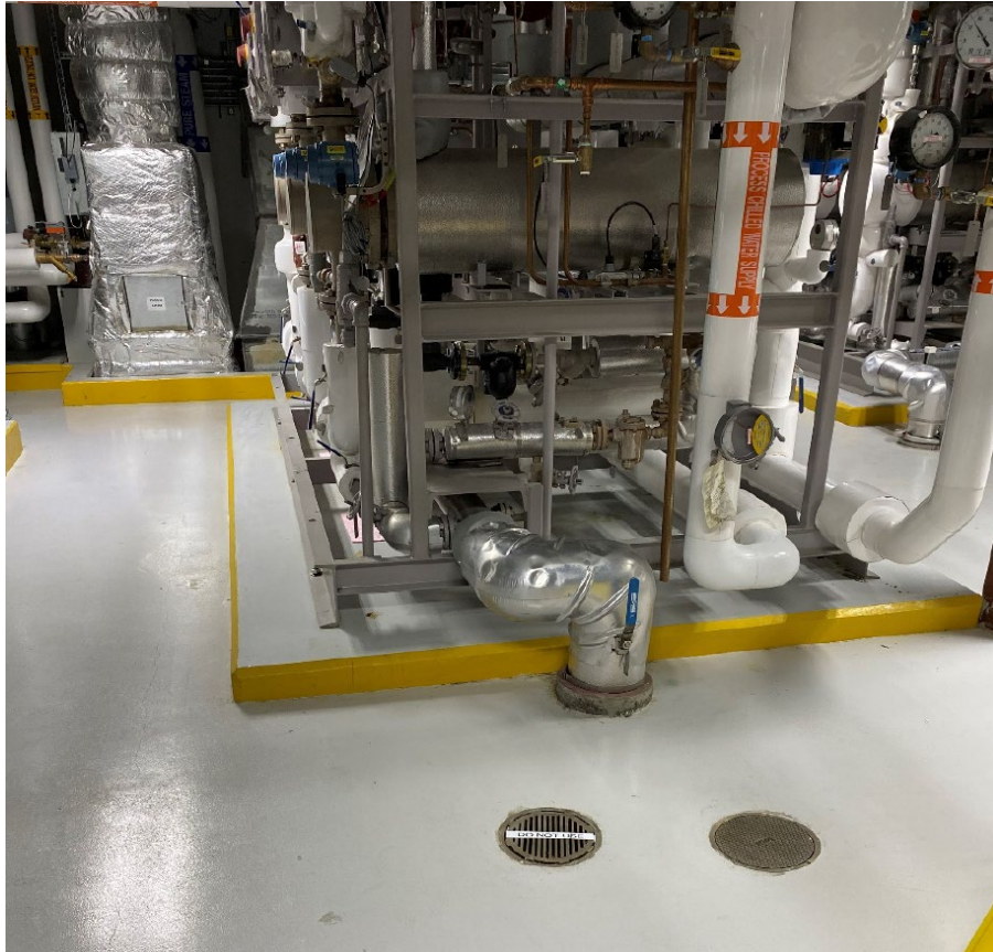
Figure 6: 7-26-22 photo of the heat exchanger and adjacent floor drain at Gilead Sciences.
