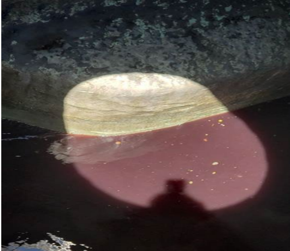
Figure 2: Burgundy-colored wastewater in MH F 0255 on August 2, 2022.
