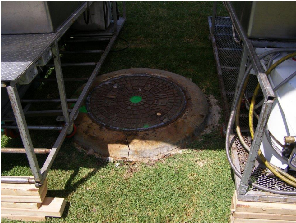
Figure 3: MH 05 0084 cover after replacement and resealing/caulking on 7-14-17.
