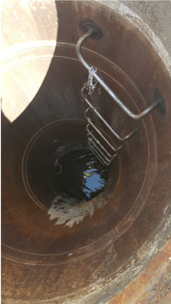
Figure 12: View into MH A 1047 on 3-27-17.
