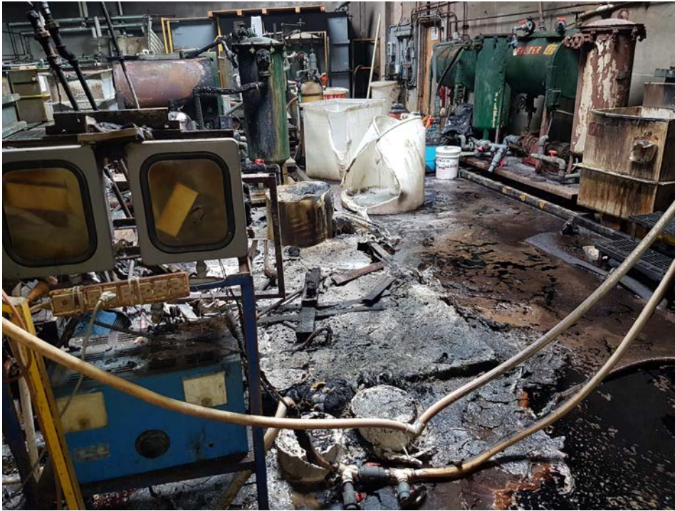
Figure 4: Aftermath of the 6-8-17 fire at Cal-Tron Plating in Santa Fe Springs. Note the melted white poly rinse tanks.
