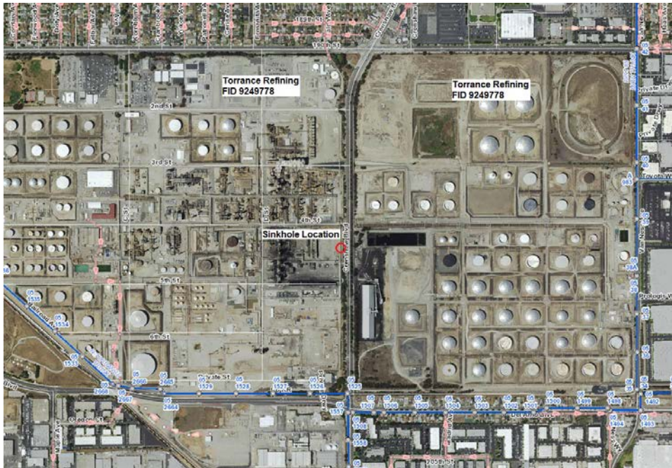
Figure 4: GIS image indicating the location of the reported sinkhole on the property of the Torrance Refining Company (formerly the ExxonMobil Oil Refinery).
