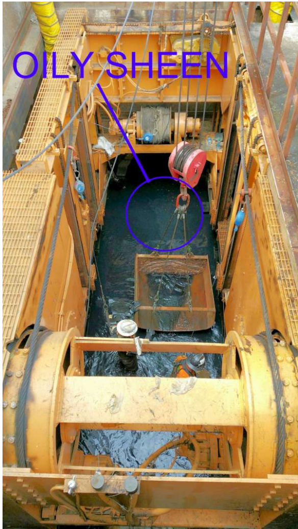
Figure 2: Sewer rehabilitation access point near MH 03A0063.
