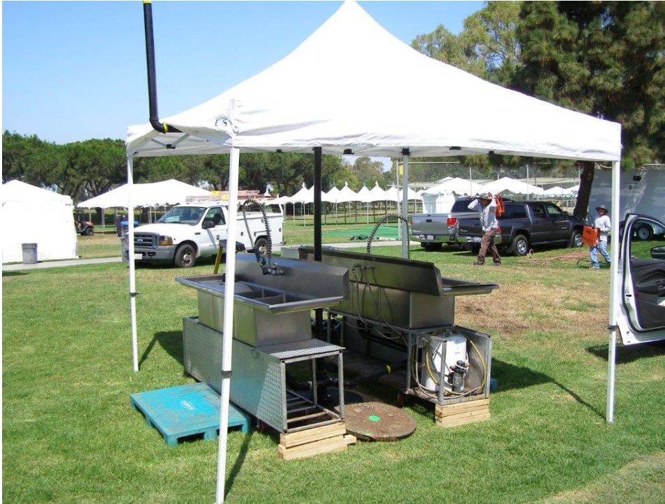
Figure 2: 7-14-17 dishwashing sinks illicitly plumbed into MH 05 0084. Note that the installation even included a vent pipe!
