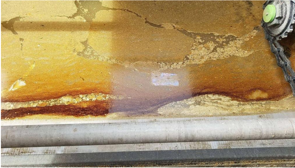
Figure 6: Floating brown oil in the Saugus WRP primary tanks at 0930 hours on 4-25-17.
