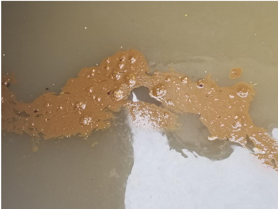
Figure 2: Brown oil in the primary tanks at Saugus WRP on 11-19-18.
