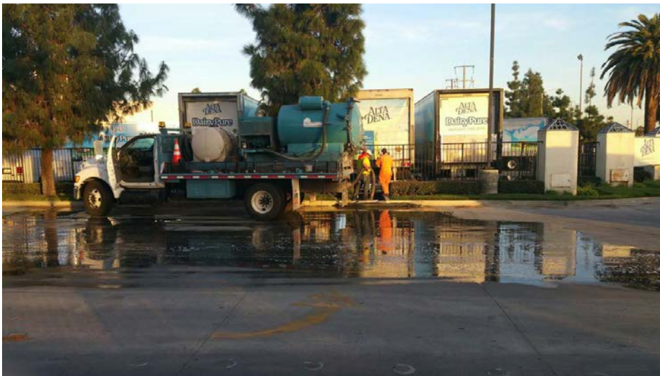
Figure 5: United Stormwater Inc. vacuum truck removing spilled wastewater from a storm drain on Valley Boulevard in front of the Alta Dena facility on 1-24-18.
