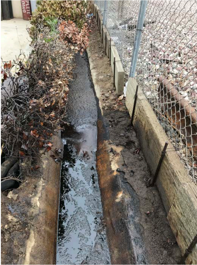
Figure 1: 10-29-18 photo taken by Inspector Finn of the oily residue from the spill. Note that its appearance matches that of the locally produced crude oil. The brine/oil came out of the ground from the broken underground line at the “hole” under the bush seen on the left side of the photo.
