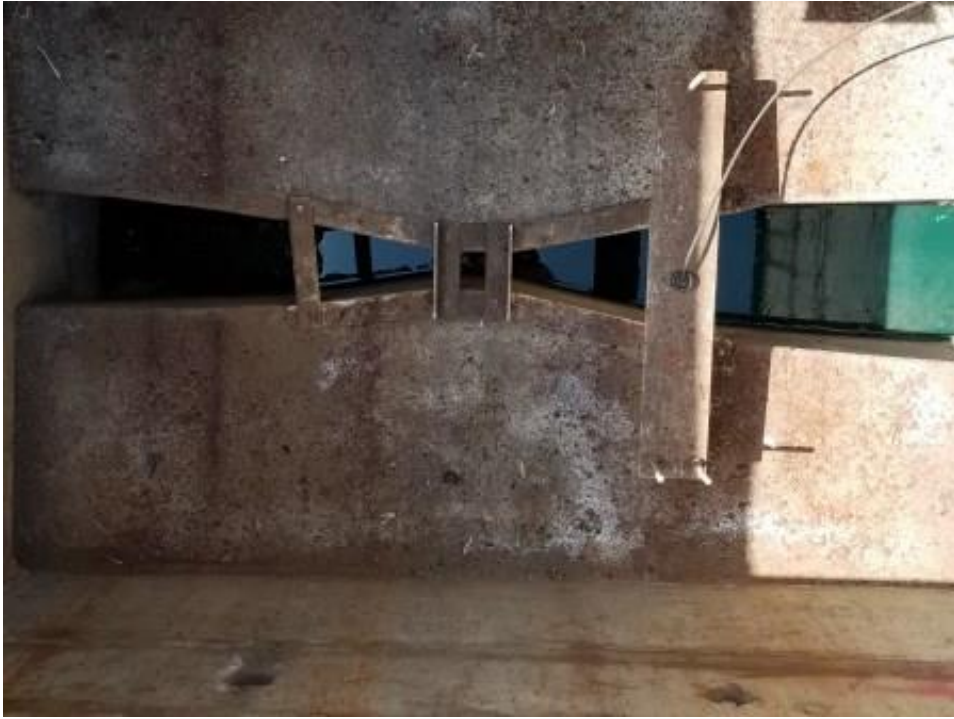
Figure 4: United Site Services residual industrial wastewater in their discharge flume on 5-10-18, note the deep blue-green color of the wastewater.
