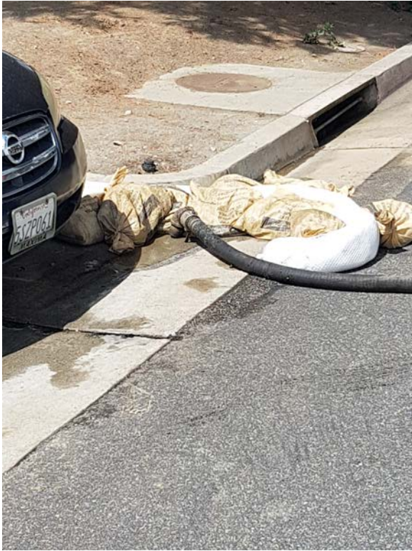
Figure 5: Street gutter sand bagging used on 5-15-18 to help keep the spilled oily brine water out of the storm drain collection system.
