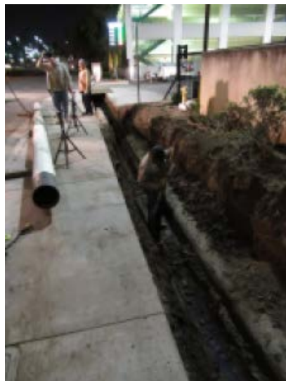
Figure 6: Installing the new pipeline.
