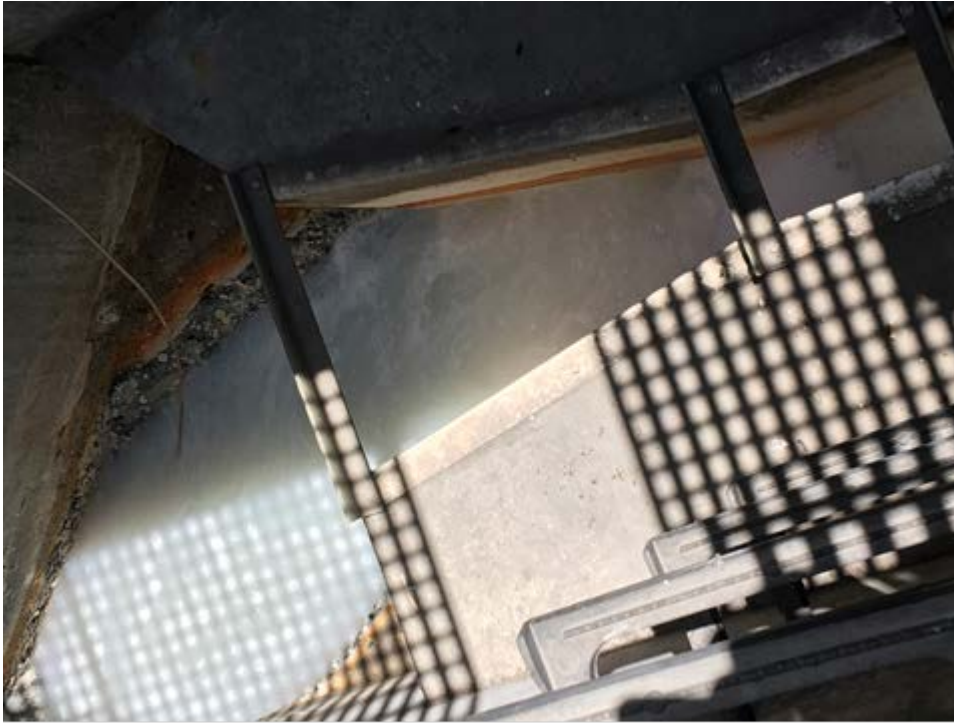
Figure 11: The industrial wastewater sampling location (tailwaters of the flume) at General Foods. Note the heavy etching present in the walls of the concrete channel immediately downstream of the fiberglass flume which indicates acidic discharges are likely occurring frequently.
