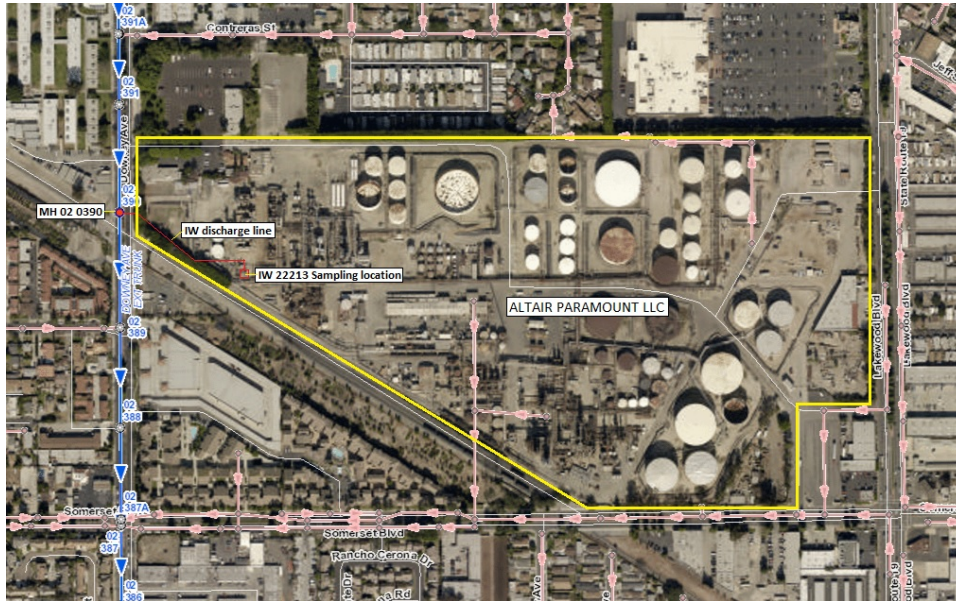
Figure 7: Annotated GIS diagram showing the relationship of the refinery, its industrial wastewater discharge line, and where it connects to the Districts' 15" Downey Ave Extension trunk sewer just north of MH 02 0390.
