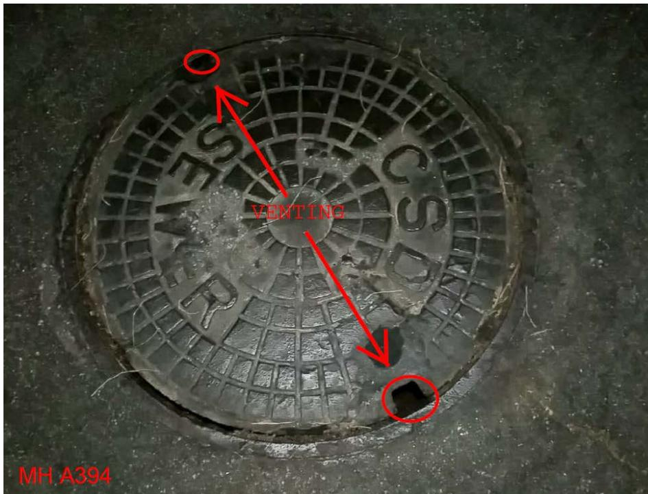
**Figure 3: 12-14-18, 1720 hours photo of MH A394. Note the open pickhole notches that were found to be venting sewer headspace gas.**
