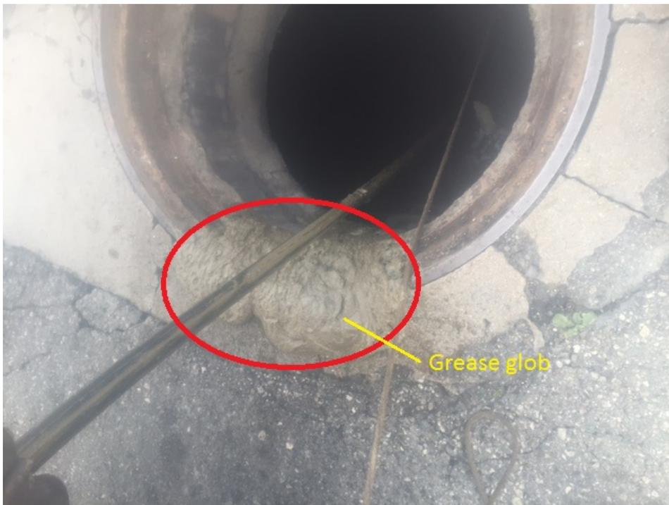
**Figure 1: Glob of grey grease removed from the 21" J.O. 'H' unit 2F trunk sewer in Vernon on 4-2-18.**
