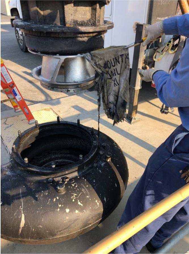
**Figure 4: 7-21-18 photo of the rag removed from the influent pump.**
