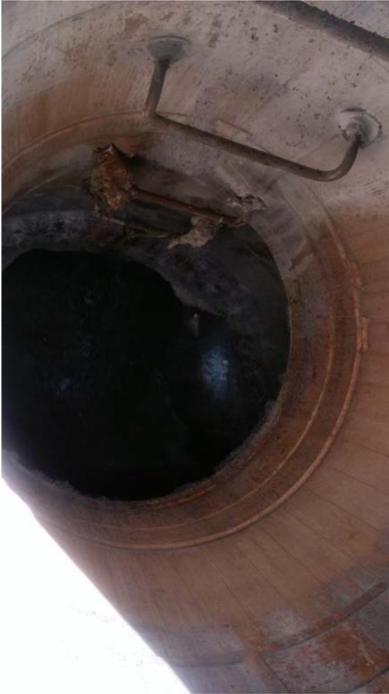
**Figure 13: 3-30-18, 1330 hour photo of the MH A1087 riser. Note that at that time only a small residual of the white foam remained on the manhole shelves. In order to escape through the pick holes it must have completely filled the riser earlier.**
