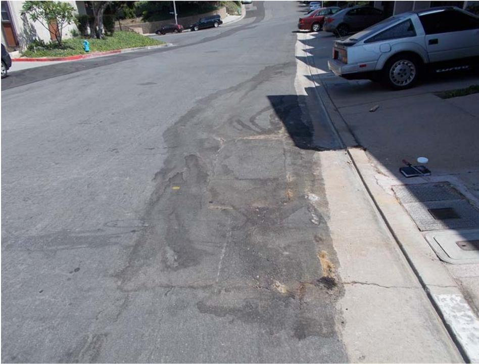
**Figure 2: Photo taken on 6-26-18 by Finn of the street cracks with whitish/yellowish powder residue in the asphalt where he noted the odorous (sulfide) gas was emanating. Note the staining indicating that either some liquid is also coming out or that someone is periodically washing down the area.**
