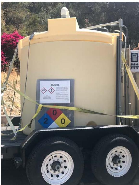
**Figure 7: 8-24-18 photo of the 750-gallon poly tank of "Bioxide" solution at the Meritage Homes' development sewer lift station.**
