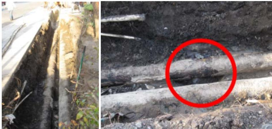
**Figures 4 and 5: Excavated pipeline and small hole in the pipeline that was the source of the leak/spill.**
