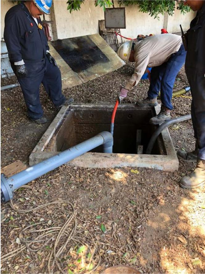
**Figure 2: Contractor jetting the line scale at the AltAir Paramount facility's private lateral line on 7-17-18.**
