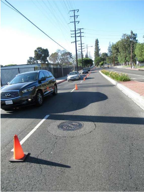
**Figure 8: 6-13-18, 1756 hours MH 02 0390 on the 15" Downey Ave. Extension Trunk. Note traffic diversion set up by Woods and McIntosh to check the line.**
