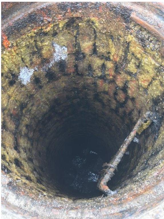
**Figure 5: MH 08 0150 riser on 3-14-18. Note the layer of biological slime growth.**
